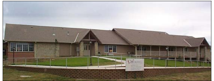
Construction of an addition/assisted living facility at the Mid-America Health Care nursing home in Lincoln was one component of the Lincoln County Comprehensive Development project.
