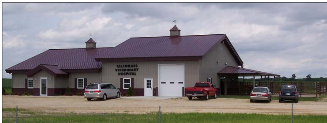
The new Tallgrass Veterinary Hospital is located north of the City of Concordia along U.S. Highway 81.
