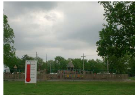
While not a direct recipient of NCK RBDTC funds, the City of Clay Center’s Dexter Park did receive a face lift following the demolition of the Swift Building. The previously hazardous structure neighbored this park for many years.
