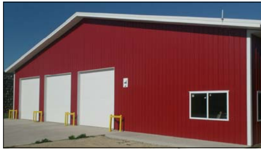
The Dickinson County Fire District 1 Station was recently constructed with volunteer labor in Woodbine as a result of a KAN STEP grant.
