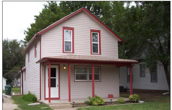
The two photos above are an example of a "Before" and "After" from a recent CDBG Housing Rehabilitation project in the region.
