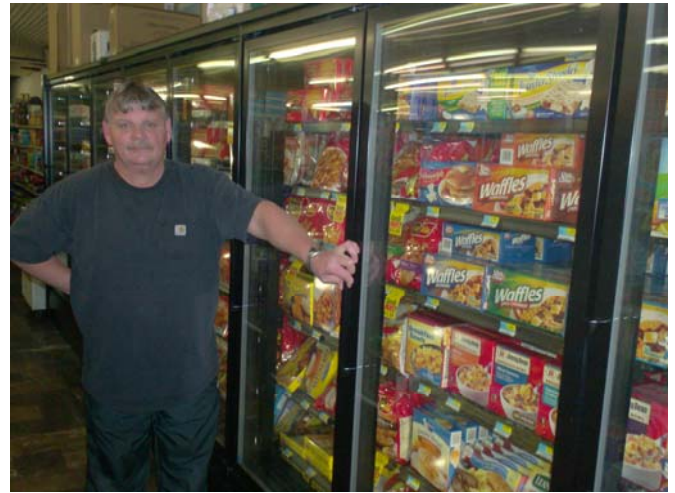
Kenny Bush, owner of Bush's Market, is pictured in front of the new energy efficient freezer unit at his grocery store. Bush's Market is located along U.S. Highway 40 in Solomon.
