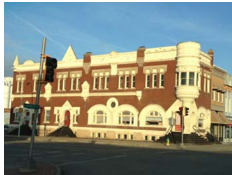
The Bankers Loan and Trust Company Building located at 101 East 6th in downtown Concordia also will be repaired with funding from the recent CDBG award.
