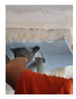
Blow insulation into cavities to density appropriate for chosen material
