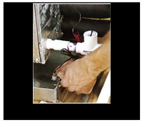
A float switch should be installed to prevent overflow and damage
