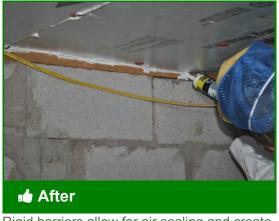
Rigid barriers allow for air sealing and create cavities for insulation
