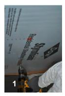
Securely fasten rigid barrier, aligning seams with joist when possible
