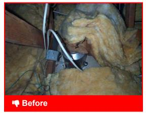
Non-IC recessed light fixtures produce excess heat and can be a fire risk
