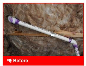
Once drainage pipes cross into unconditioned space, they can freeze
