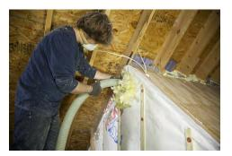
Insulation should meet manufacturer specifications for density.
