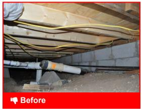
Crawl spaces lacking moisture barrier risk moisture penetration of floor
