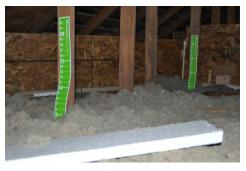
Install depth markers and insulation dams above height of insulation
