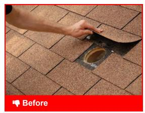
Holes for termination fitting need to be sealed to weatherproof
