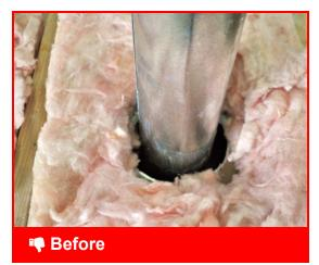
Gaps and penetrations in attic need to be sealed to maintain air barrier
