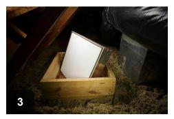
Weatherstrip around bottom edge of hatch cover to create air tight seal
