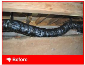
Ducts should not be allowed to droop and drag, adding distance to run
