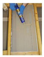
When supporting from above, apply adhesive between drywall and bracing
