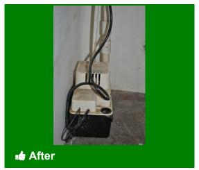
For non-gravity draining systems, a pump is necessary
