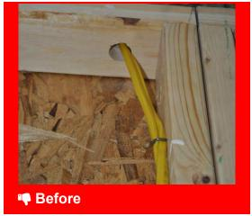
Penetrations and bypasses create places where blown in insulation can leak
