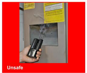
Test natural draft furnace or water heater for spillage in excess of 2min
