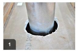
Prepare work area by removing any insulation and debris
