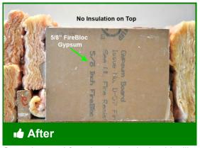
Once dammed from insulation, it should still not have insulation on top
