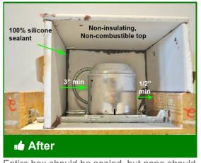
Entire box should be sealed, but none should come in contact with light
