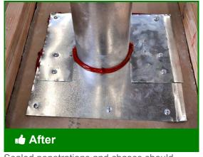
Sealed penetrations and chases should utilize high-temperature materials
