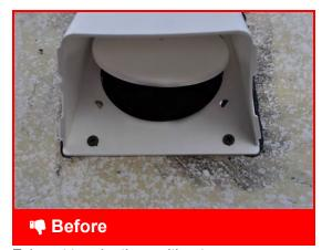
Exhaust terminations without screens are an invitation to pest intrusion
