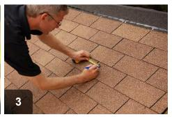
Based on termination fitting size (in this case, 4"), mark to cut hole
