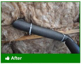
Pipes in unconditioned spaces should be insulated with 1" pipe insulation
