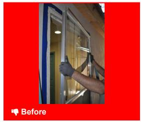
Single pane window is being removed to install double pane unit
