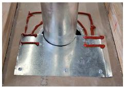
Metal sheeting should be used to construct seals and dams on flues
