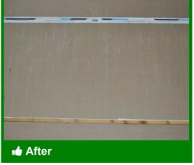
Rigid material encloses the soffit into the conditioned living space
