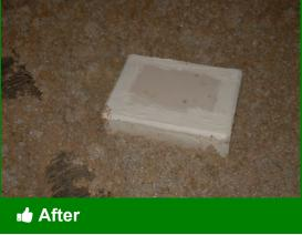
Sealed box around non-IC light should be taller than surrounding insulation
