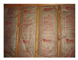
OR: Wall can be insulated using batts installed without gaps
