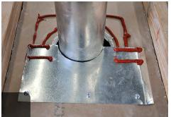
Fasten rigid material (metal sheeting) and apply additional caulking
