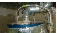
Inspect for missing draft diverter
