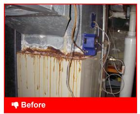
Damaged combustion appliances beyond repair should be replaced
