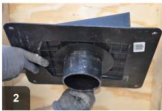
Termination fittings with collars should Collared fittings extend through the be used for exhaust ventilation
