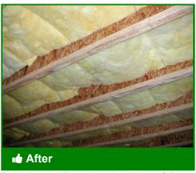
"Lightning rods" or twine should keep full contact with the subfloor
