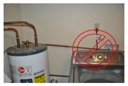
BAD: T&P discharge should not be piped into drainage system
