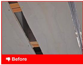
With rigid block in place under bonus room stem wall, insulation can begin
