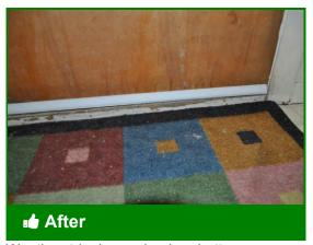
Weatherstripping and a door bottom minimize air infiltration around doors
