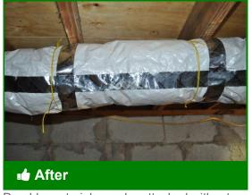
Durable materials can be attached without compressing insulation
