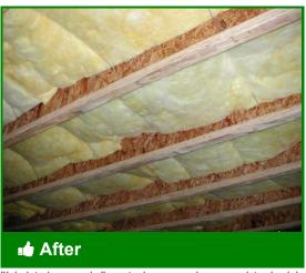
"Lightning rods" or twine can be used to hold batts in contact
