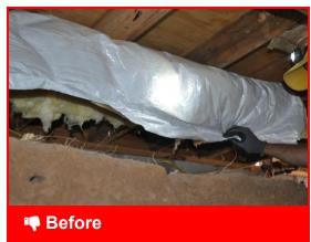
Unsecured and sealed insulation around ducts is useless
