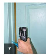
Check interior doors for pressure differential either using smoke pencil or hand
