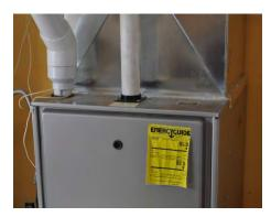
Two-pipe 90% efficiency furnaces are viable replacement appliances
