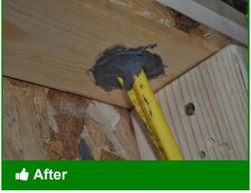
Sealed penetrations offer leakage protection and keep insulation in place
