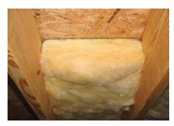
Batt should be in contact with subfloor without being compressed
