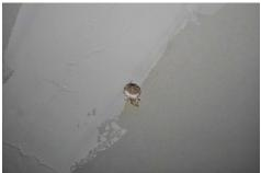
Cut small test holes in cavities to verify specified density has been met
