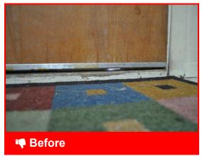
Daylight visible around door can indicate it does not hang true and leaks
