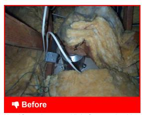
Non-IC rated recessed light fixtures should be dammed from insulation
