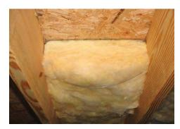
Batts should have full contact with subfloor without being compressed
