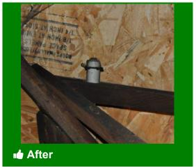
Knob and tube wiring may get hot and cannot If possible, k&t wiring should be disabled and replaced with modern wiring
