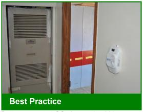
Battery operated CO alarms should be UL-2075 or UL-2034 compliant
