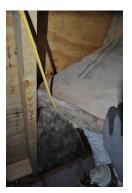
Install kraft-faced batts with paper against subfloor
