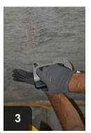
Keep netting taut while stapling to prevent wrinkles and leakage
