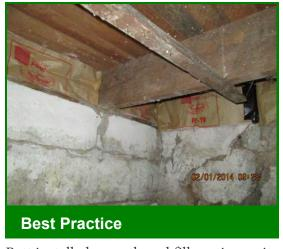
Batt installed smooth and fills entire cavity
