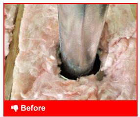
Gaps around combustion exhaust flues need to be sealed
