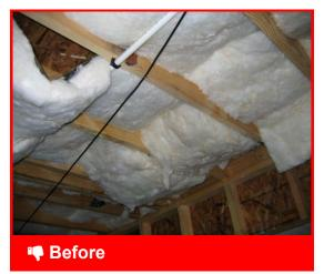
Insulation should be secured to prevent drooping or movement
