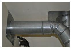
Inspect ventilation systems for inadequate slope
