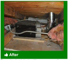
Properly sized ducts with snug connections to collared fittings last longer
