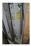
GOOD: T&P discharge should be piped within 6" of the floor or to outdoors
