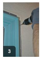
Flanges have been folded out to allow Fasten window flange securely around exterior of entire window
