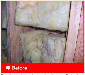
Existing batt insulation should be adjusted to fit properly
