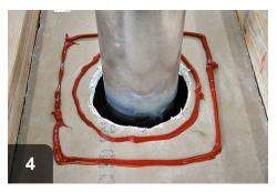
Apply second ring of caulking to size and shape of rigid material
