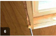
Fill interior gap with compressible foam or appropriate sealant
