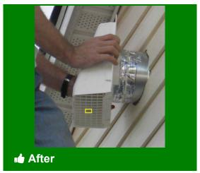
Screen mesh should be between 1/4" and 1/2" in either direction
