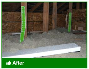
Depth markers and insulation dams aid in proper insulation of attic spaces
