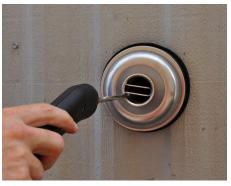
Test accessible exhaust outlets for direct-vent appliances
