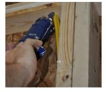
Seal penetration with caulk or fireblock, as appropriate
