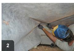
Secure netting across sills to prevent leakage of insulation
