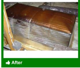
Insulated pull-down stairs cover installed to prevent air leakage
