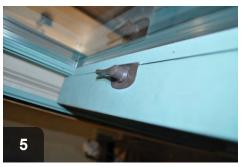
Check that sash locks align properly, indicating window is plumb
