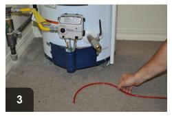
Place test hose by combustion appliance
