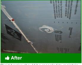
Rigid barrier should be resealed to maintain air barrier after filling
