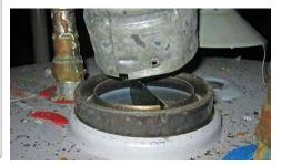
Inspect ventilation systems for disconnected pipes
