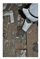
Check cavity for electrical junction and flagged electrical penetrations
