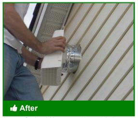
A snug fit should be ensured to minimize weatherproofing required
