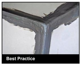
Sealants, like mesh and UL 181 mastic, meet IRC, ASTM, and UL specs
