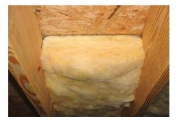
Ensure batts are in full contact with subfloor and remain uncompressed
