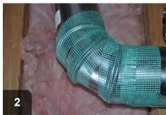
Wrap joint with fiberglass mesh tape
