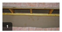
Soffits open to the attic need to be sealed to maintain air barrier
