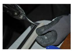
Notch upper ends of side weatherstripping to allow for top piece
