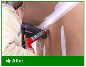
Seal penetrations to minimize risks and air leakage
