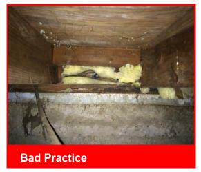
Compressed batt insulation in Rim Joist
