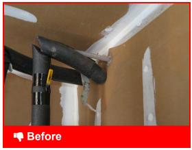
Penetrations between the garage and house can leak hazardous fumes
