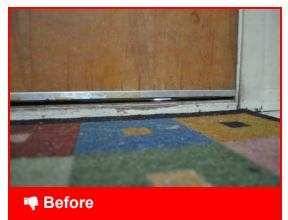
Daylight visible around an exterior door indicates air infiltration
