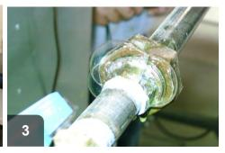
If bubbles develop, leak is present. Notify occupant
