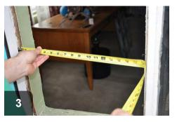
Cut replacement glass 1/8" smaller than measured opening
