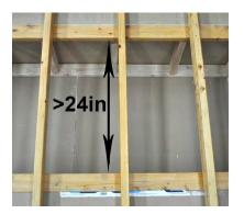
Create bracing to support spans larger than 24", either from above or below
