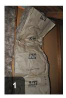
Where existing insulation is improperly Kraft-face should go to "warm in installed, fix it
