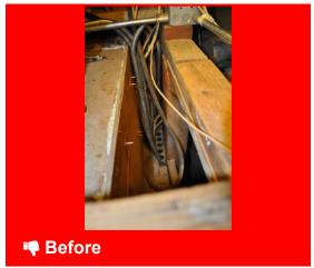
Chases need to be capped and sealed to prevent leakage
