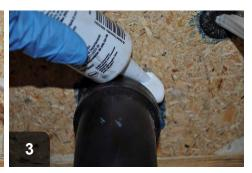
Apply appropriate caulking to ensure backing/infill does not move
