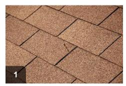
Locate the center of your vent hole by drilling from inside through roof
