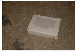
Non-IC can lights should be covered with a damn and have no insulation on top
