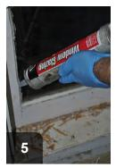
With push points in place, glaze to air seal new glass pane in sash
