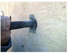
For stucco and plaster patches, lath will need to be used to hold weight
