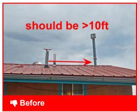
Exhaust vent has been improperly mounted too close to mechanical vent
