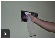
Wet the edges of the drywall to ensure a good bond
