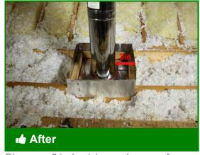
Observe a 3 inch minimum clearance for dams around flues and chimneys
