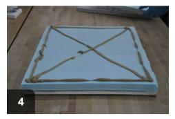
Repeat adhesive and XPS layers to reach maximum R-value without making hatch excessively heavy or awkward
