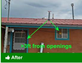
Exhaust vent was properly mounted over 3ft from door, window, and deed line
