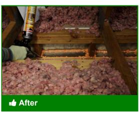
Wall cavities capped and air-sealed in one of a variety of options
