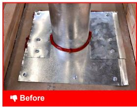
To prevent fire hazards, flues, chimneys, and light fixtures require dams
