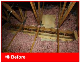
Accessible drop soffits should be sealed to prevent heat gain/loss
