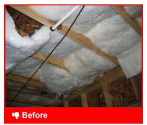
Fiberglass batts should not be hanging away from subfloor
