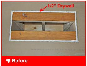
Unsealed standard chases covered with drywall can be leakage points
