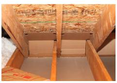
Baffles should be securely fastened to Once baffles are properly installed, insulation can be placed against them
