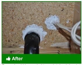
Gaps should be sealed to maintain air barrier
