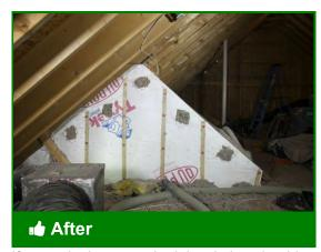
If properly dense-packed, insulation should hold in place when finished
