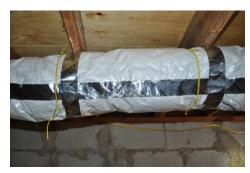
Ducts in unconditioned areas should have r-8 insulation with vapor barrier
