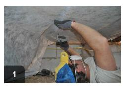
Secure netting across each joist to create separate cavities
