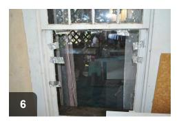
Secure pane in place with tape to hold until glazing sets
