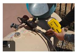
Check all raw fuel lines for leaks
