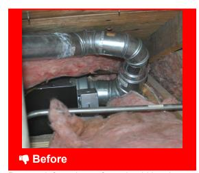
Duct work for exhaust fans should be short, smooth, and not pinch down
