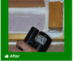
Whatever option chosen, test for visible air movement with smoke pencil
