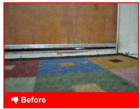
Daylight visible under exterior doors indicate water can leak in
