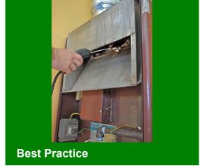
Test CO levels in undiluted flue gases and exhaust outlets, when accessible
