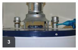
Retest spillage after repairs have been completed to verify problem has been corrected
