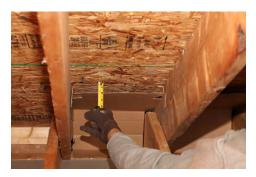
Allow a standard two inch gap for air flow through eave
