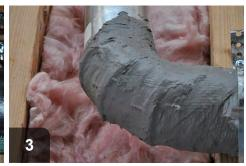
Apply UL 181 mastic to seal joint
