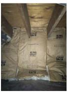
Cutt Batts to fit around joists.
