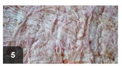
Insulate over now-capped soffit
