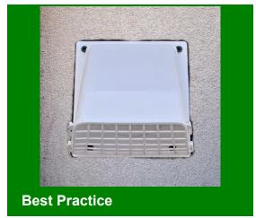
Termination fittings for dryers should have backdraft dampers
