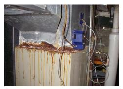
Assess existing combustion appliances for damage and replace when necessary
