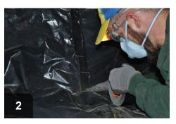
Tape (overlapped) floor seams to prevent movement and water leakage
