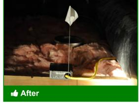
Flag electrical junctions to make future maintenance and repairs easier
