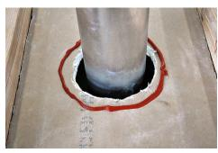
High temperature caulk should be used for flues and chimneys
