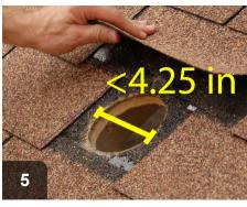
Verify hole size is correct before installation
