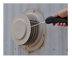
Test accessible exhaust outlets for power-vented appliances
