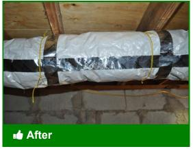
All seams should be sealed with UL-181 duct tape to preserve vapor barrier
