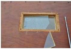
Remove broken glass and clean old sealant and glazing from rough opening
