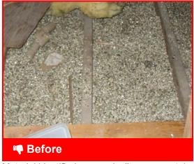
Material identified as vermiculite may contain asbestos
