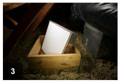
Build dam to hold back attic insulation Weatherstrip underside of hatch cover to create tight seal
