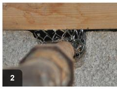
In holes larger than 1/4 inch, wire mesh should be used for backing
