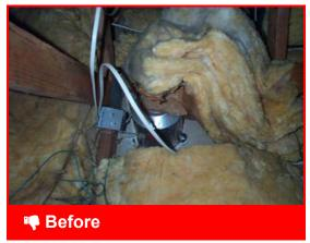
Non-IC rated recessed lights produce excess heat and can be a fire risk
