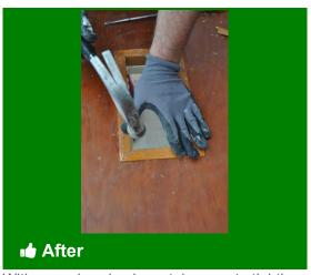
With new glass in place, take care to tightly seal and replace stops
