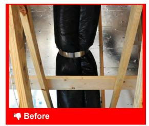
Materials holding insulation in place should not compress or kink duct
