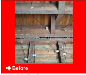
Live knob & tube wiring may get hot and should not be insulated over
