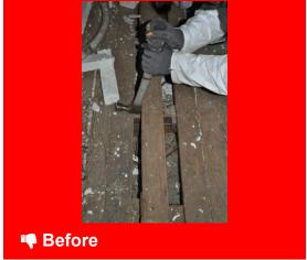
Remove flooring in attic spaces to access floor cavities and insulate
