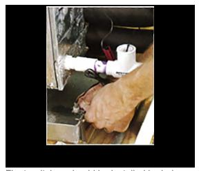
Float switches should be installed in drainage pans to prevent overflow
