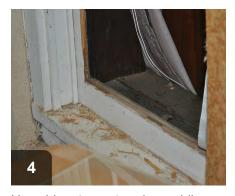
Use shims to center glass while installing push points
