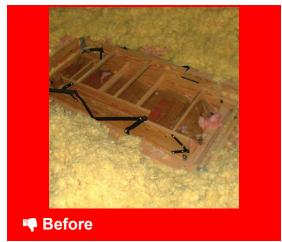
Insulation needs to be dammed to keep from falling through during operation
