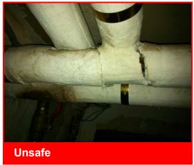
Suspicious pipe insulation may contain asbestos
