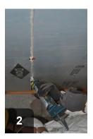
Seal all seams with caulk to prevent leakage
