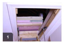
Stairs and hatch should both be insulated to match r-value of attic
