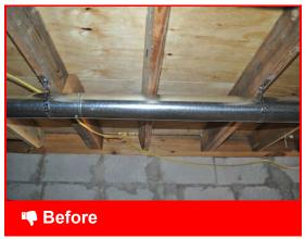
Uninsulated ducts in unconditioned spaces are an energy drain
