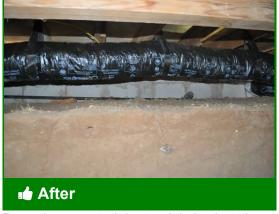
Properly supported ducts minimize heat loss and and maximize duct run
