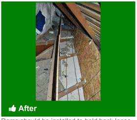
Dams should be installed to hold back loose fill insulation
