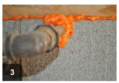
Cement or caulk exterior holes. Foam or caulk interior holes
