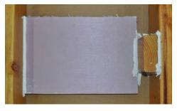
Option 3, Step 2, Option A: Cap with XPS and seal exposed joints
