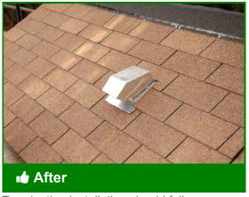
Termination installation should follow shingling to deter water penetration
