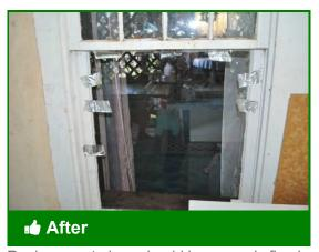
Replacement glass should be securely fixed with points and glazing
