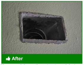
Use a mesh in mastic system to seal duct boot to interior surface
