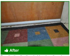
By adjusting the threshold and sealing along it, water should be kept out
