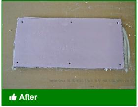
The air barrier is be maintained by capping chases with rigid material
