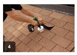
Hole should be no more than 1/4" larger than termination fitting diameter
