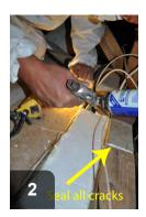
Sealant is used to fill in all cracks and Cap is sealed gaps along edges of chase cap
