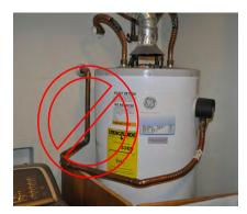
BAD: T&P discharge should flow with gravity and be observable
