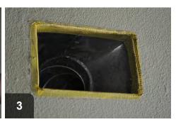
Cut mesh tape to fit around duct boot and cover gaps
