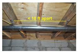
Metal ducts should be supported every Metal straps should be at least 18 10 feet or less with straps or wire
