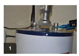
If spillage exceeds 2min, steps should be taken to correct draft issue
