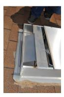
Backdraft damper on roof mounted exhaust fan
