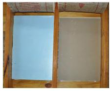
Option 1, Step 2: Cover openings with rigid material, either XPS or drywall
