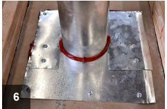
Fasten rigid material to cover penetration and seal against flue with
