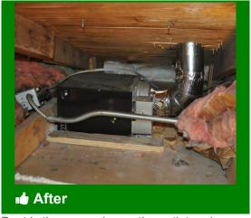
Duct is the same size as the outlet and makes shortest run possible
