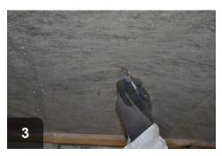
Cut holes in each individual cavity to insert insulation machine nozzle
