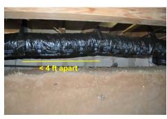
Flex ducts should have supports no less than every 4 feet
