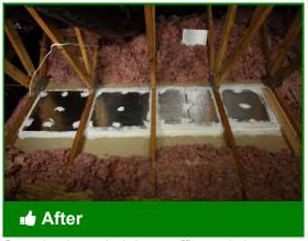
Completely sealed drop soffits and chases minimize heat transfer
