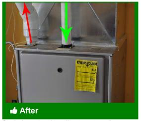
Sealed-combustion, direct-vent appliances should replace unsafe appliances
