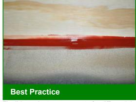
Flexible sealants compensate for differential expansion and maintain a seal
