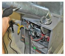
Test undiluted flue gases in induceddraft furnaces
