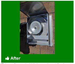
This roof-mounted kitchen exhaust fan is galvanized steel--heat resistant
