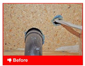
Gaps around floor penetrations, such as plumbing, HVAC, and electrical
