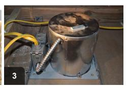
OR non-IC can light can be replaced with IC-rated recessed light
