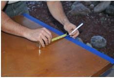
Measure and trim door, if necessary, to allow for door bottom
