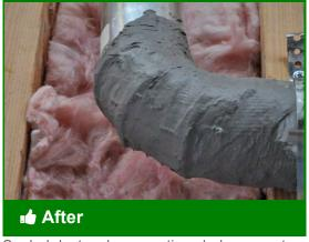
Sealed ductwork connections help prevent leakage
