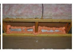
Option 2: Backing used to fill bays and sealed with spray foam
