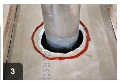
Apply first ring of caulking to match shape of opening
