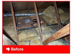
Unsealed attic hatches and panel doors allow air leakage to and from attic
