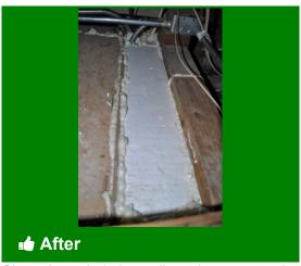
Chase is sealed along all cracks, gaps, and penetrations
