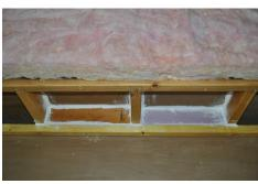
Option 1: Span each stud bay with rigid material at level of soffit
