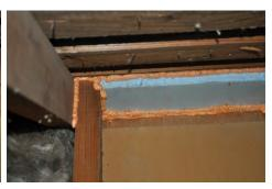
Top plate holds dense pack insulation New top plate should be sealed to surrounding joists and studs
