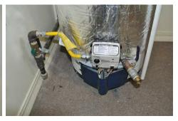
Wrap does not obstruct ventiation, thermostat access plate, hi-limit switch, or fuel line
