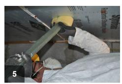
Dense pack insulation into floor cavities
