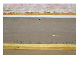
Sealing with drywall reduces overall combustibility of paneled chases
