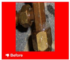
Fuel leaks need to be repaired by appropriate professional
