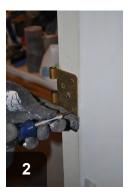
Adjust hinge plates to bring door back Adjust strike plate to allow for secure into true
