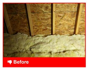
Insulation should not block vented eaves
