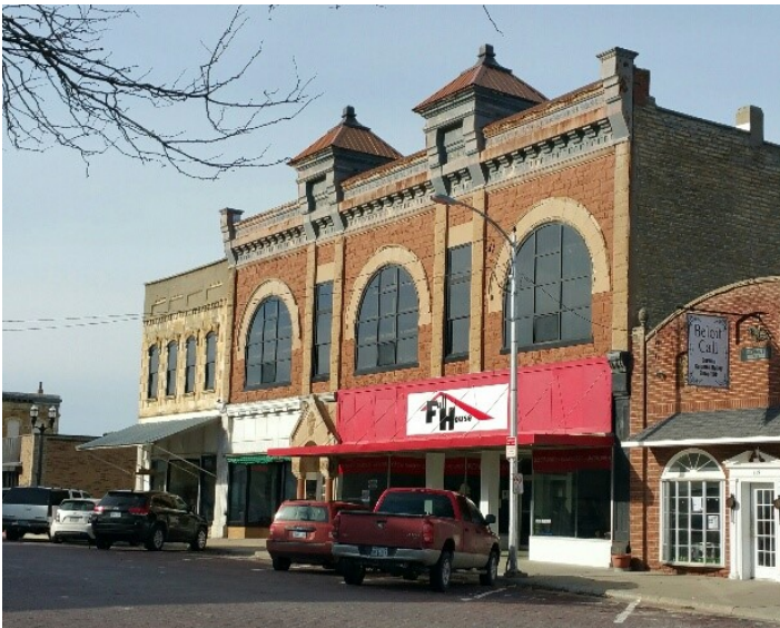
A building in downtown Beloit which used commercial rehabilitation funding to make façade, roof and structural improvements. NCRPC served as the project administrator.
