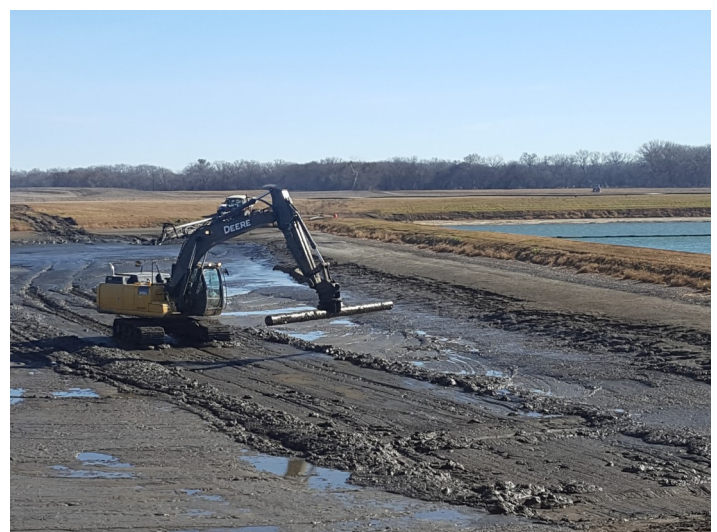
A contractor works on making improvements to the existing wastewater lagoons serving the City of Clyde. This is just one example of the many water/wastewater projects administered by NCRPC.
