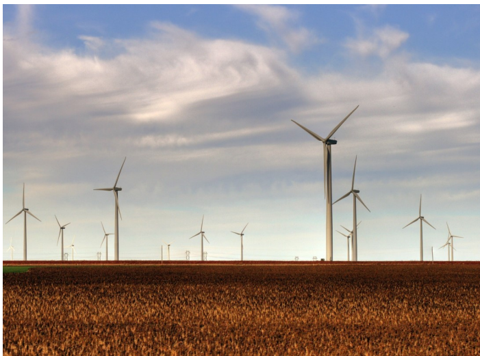
Smoky Hills Wind Farm in Lincoln and Ellsworth County
