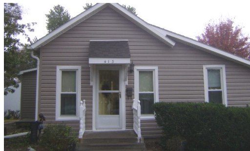
These images show a house before (left) and after (right) being renovated through the housing rehabilitation program.
