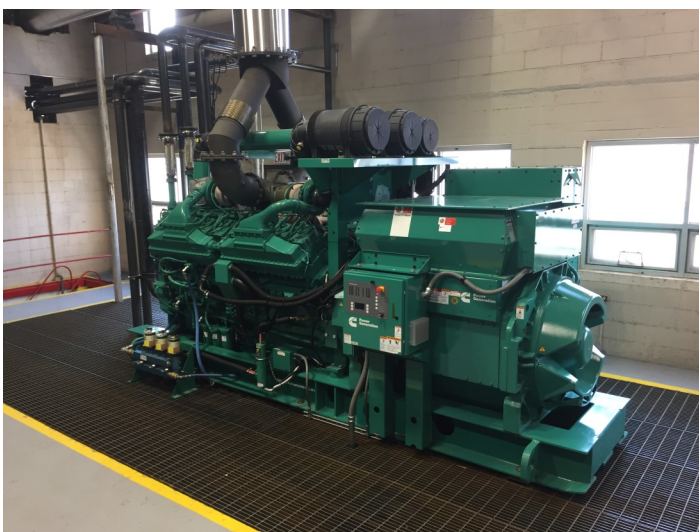
Lincoln Center City made improvements to their city power plant by purchasing and installing a new generator. This is just one example of the many community facilities projects administered by NCRPC.
