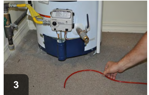
3 Place test hose by combustion appliance
