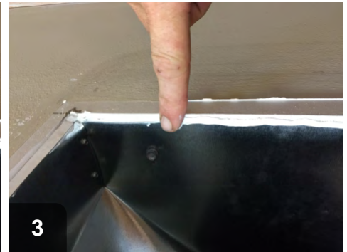
Wipe the caulk into the joint and smooth it as you go
