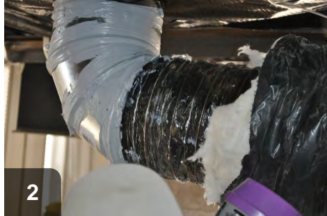
2 Slide inner liner onto flange with sealant
