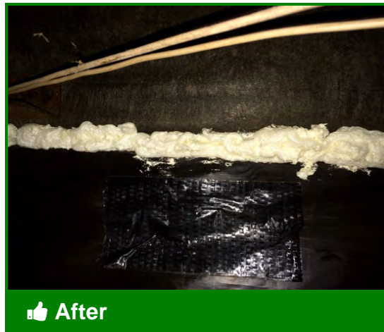
Completed air sealing at marriage line
