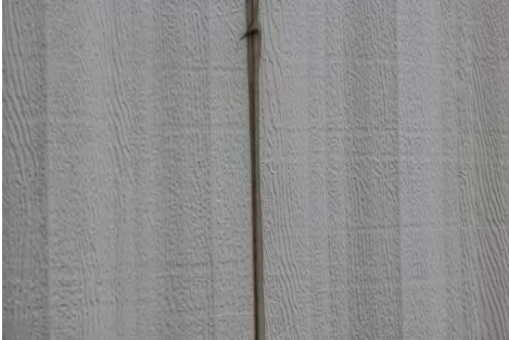
Seams on aluminum siding must be tight.
