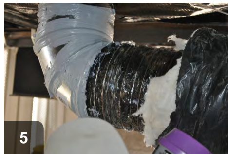
5 Slide inner liner onto flange with sealant
