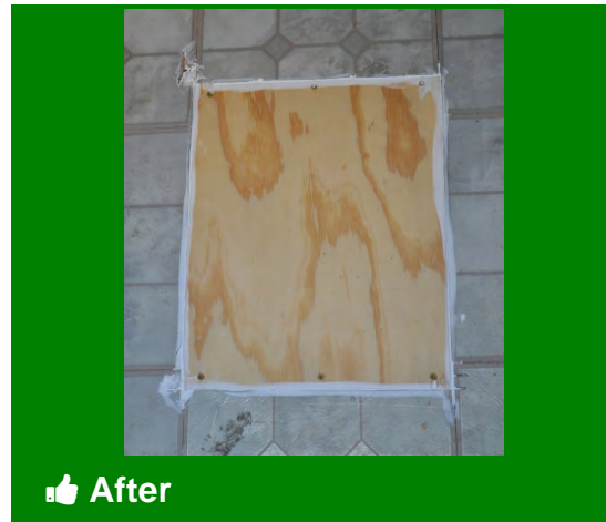
Completed floor patches should be air sealed to prevent leakage from belly
