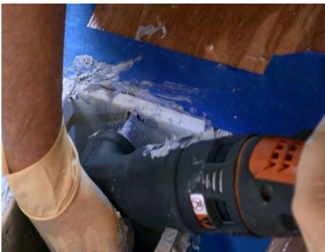
Mechanically fasten the boot to the subfloor.
