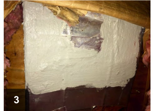
3 Overlap foil tape with mastic by at least one inch on all sides
