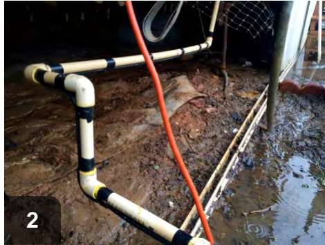
2 Fasten heat tape to pipe with electrical tape every six inches.
