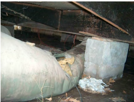
Removing the crossover duct may provide access to the plenum. Replace and seal the crossover duct after sealing plenum
