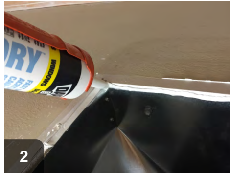
Caulk the boot to the gypsum board. Angle the tip forward and force caulk into the joint
