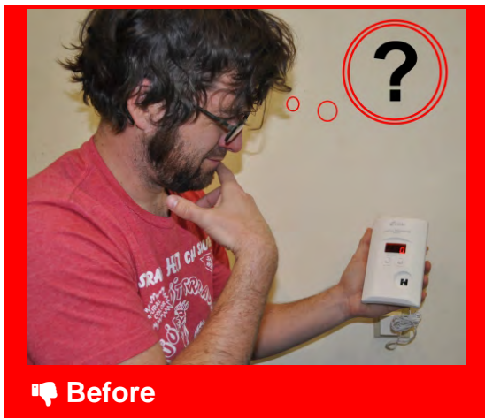
Before Occupants may be unfamiliar with CO alarms and proper operation and maintenance
