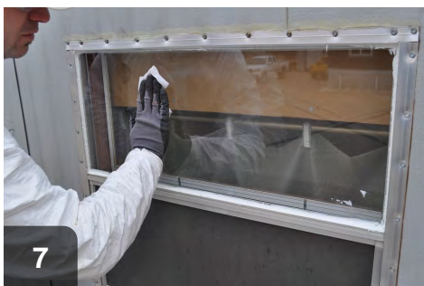
7 Clean glass to ensure than no out of place adhesive or glazing remains to bake onto glass
