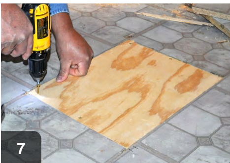
7 Securely fasten new subfloor in place, attaching to joist or blocking as necessary
