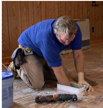
Fit the new boot on to the trunk line.
