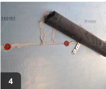
4 A rigid air barrier should be securely in place so prevent sagging, gaps and penetrations should be sealed
