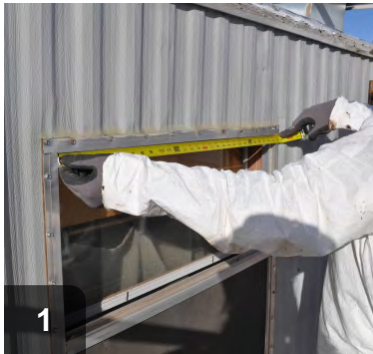
1 Measure sash for width of replacement glass -- cut glass to 1/4" less than sash width
