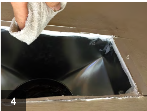
Wipe away excess caulk (use water on siliconized acrylic, alcohol on silicone, and solvent on polyurethane caulk)
