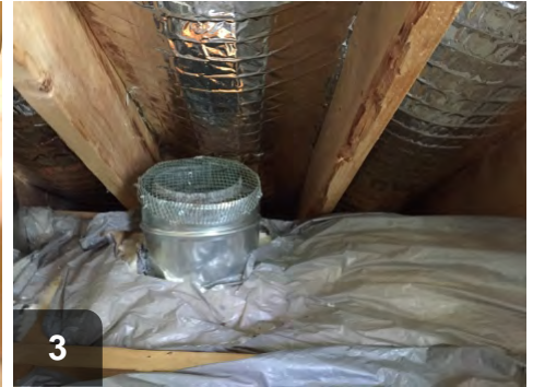
Fasten 1/4" galvanized hardware cloth over high/low vent openings
