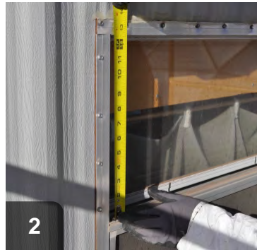
2 Measure sash for height of replacement glass -- cut glass to 1/4" less than sash height
