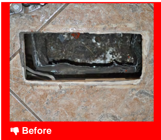
Unattached ducts are useless
