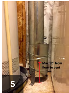
Terminate the low vent within 12" of the floor. This one is mounted inside a section of larger diameter metal duct
