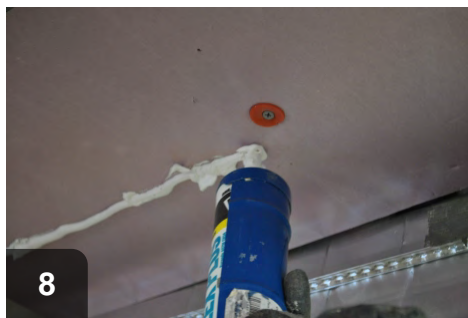
8 When insulating around low-hanging ducts and water pipes, run a line of sealant before placing insulation
