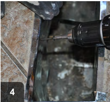
4 Use metal fasteners to secure duct to subfloor
