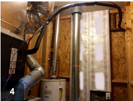
Complete installation by adding supports and fasteners as required for stability and durability
