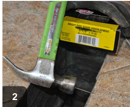
2 Use ring-shank nails to hold ducting in place to subfloor
