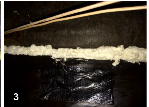
3 Apply foam or caulking over backer
