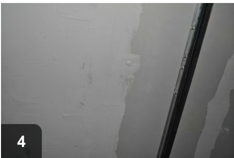
Add joint tape and first coat of joint compound
