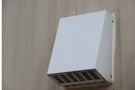
Through the wall exhaust fan sealing.
