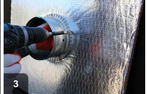
3 Fasten the collar to the backer ring by driving at least three equally spaced screws through the collar, duct board
