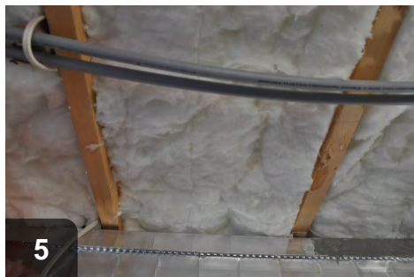
5 When ductwork or water pipes run below joists, insulation should be threaded above to fill joist cavity, uncompressed
