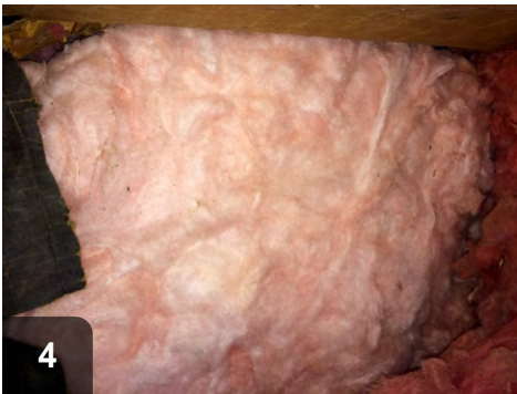
4 Replace or reinstall fiberglass belly insulation
