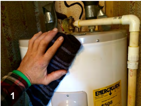
1 Clean the entire outside of the water heater
