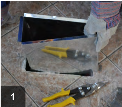
1 Replace damaged ducting if necessary
