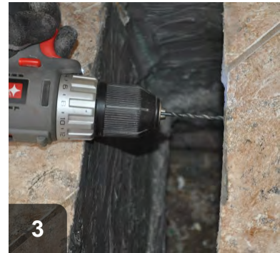
3 Drill pilot holes for metal fasteners
