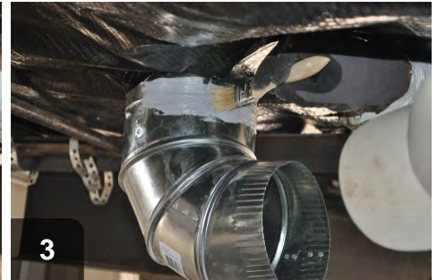
3 Apply mastic at metal-to-metal connection
