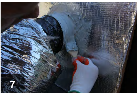
7 Coat seam with mastic
