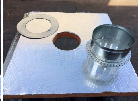
Select starting collar with tabs matching the thickness of the duct board
