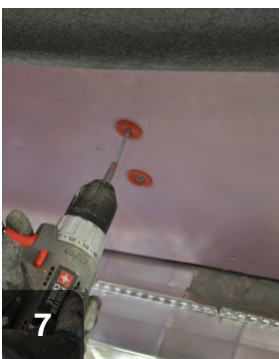
7 A rigid air barrier should be mechanically fastened to hold it tight against the floor joists
