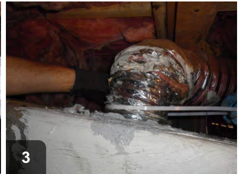
3 Install duct liner onto collar and secure with properly tensioned zip tie
