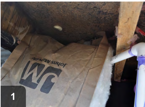
1 If fiberglass insulation is kraft-faced, ensure kraft is in contact with subfloor
