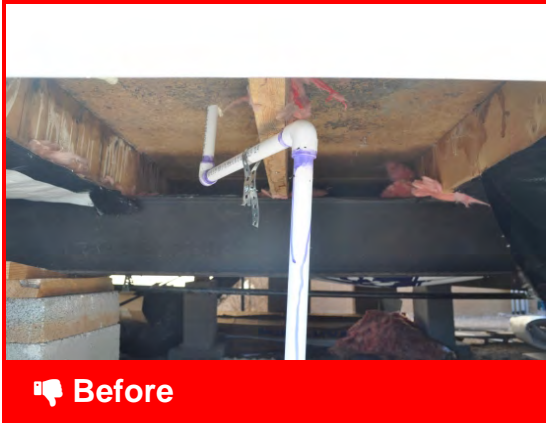
Uninsulated floors over unconditioned spaces are an energy drain
