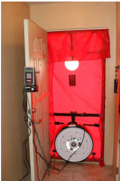
Set-up blower door to perform pressure pan testing. Depressurize to -50 pascals
