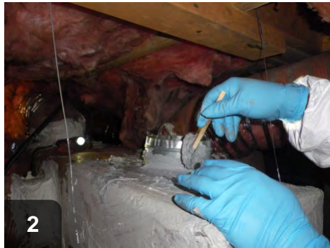
2 Apply mastic to metal collar
