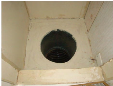
Apply mastic to inside seams of plenum
