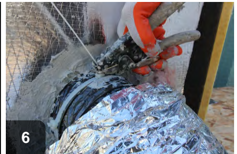
6 Secure with properly tensioned zip tie.
