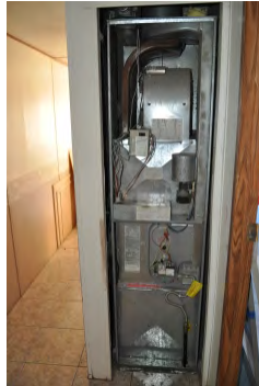
Test undiluted flue gases in induced-draft furnaces
