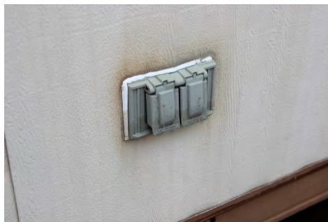
Exterior electrical outlet sealing.
