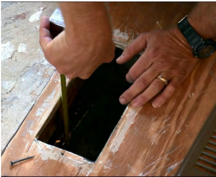
Measure the dimensions required for the new boot.
