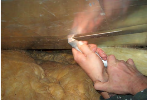
Cut belly to expose duct trunk. Use a utility knife to cut access under furnace plenum
