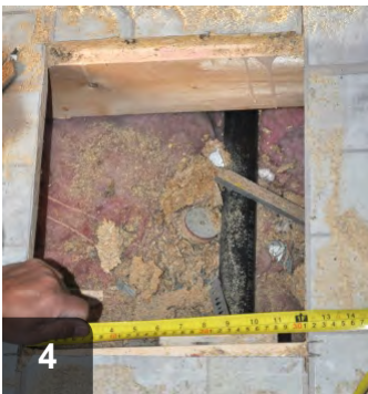
4 Once damaged area has been removed, measure for new patch and cut replacement subflooring to size
