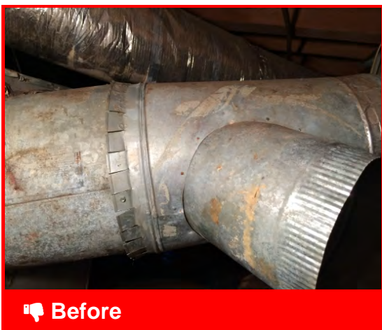
Unsealed metal ductwork
