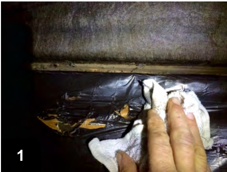
1 Clean belly wrap before air sealing
