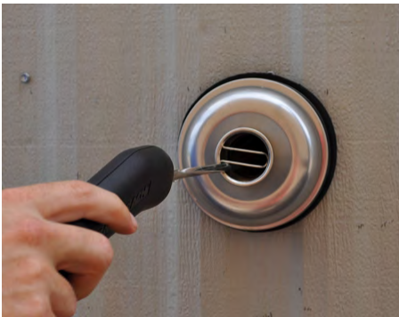
Test accessible exhaust outlets for power-vented appliances
