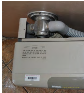
Ensure new combustion appliances are vented properly
