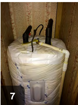
7 Use remaining insulation for the top of electric water heaters. Tape up seams in the vapor barrier. Insulate water lines
