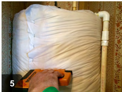
5 Staple the flap to the blanket with outward clinching staples or use long zip ties to secure the blanket in place
