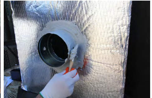
Apply mastic liberally and install flex duct
