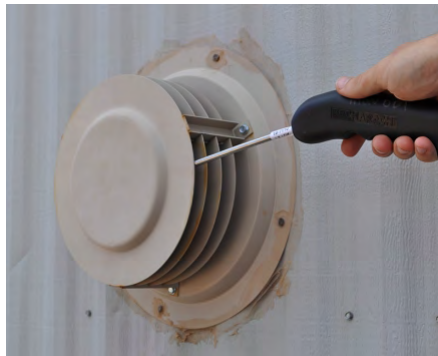
Test accessible exhaust outlets for direct-vent appliances
