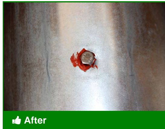
The hole in both walls has been properly sealed with a plug, cap, or other approved method.
