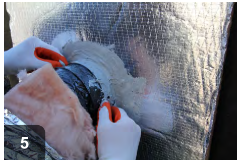
5 Slide flex duct liner over mastic-coated metal collar
