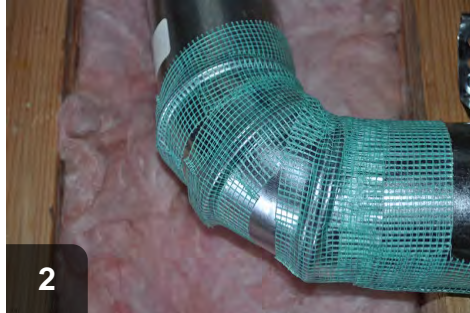
2 Wrap joint with fiberglass mesh tape
