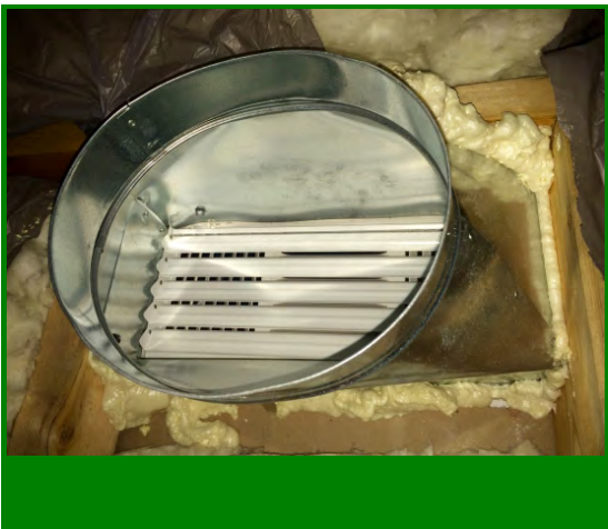
Register boot fastened to framing and sealed to gypsum with spray foam
