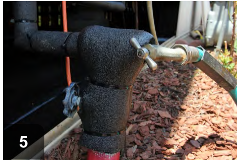
5 Cover all exposed portions of the water supply lines with insulation
