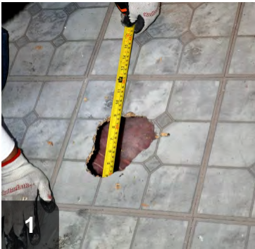
1 When possible, measure patch to reach surrounding joist. If not, blocking will be required.
