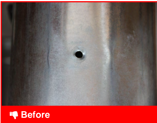
The testing hole was left unsealed.
