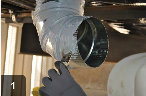
1 Apply mastic to flange
