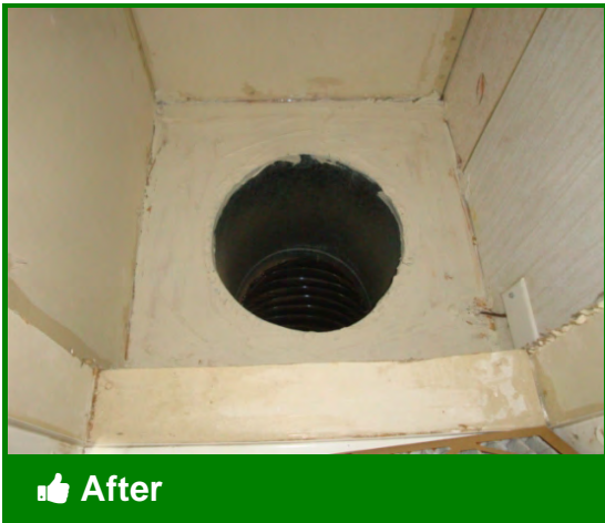
Closet prepared for furnace installation
