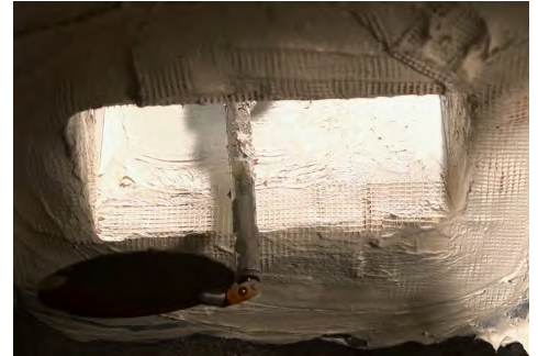
Seal the boot to the trunk line using mastic and mesh tape. An inspection mirror can make this easier.
