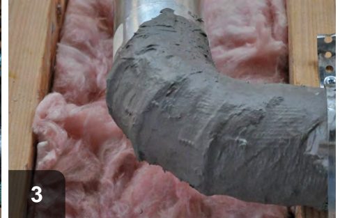
3 Apply UL 181 mastic to seal joint
