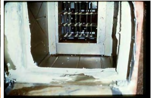
Using mastic and mesh tape, fully seal the furnace to the trunk line. Repair and seal the access holes in duct and belly
