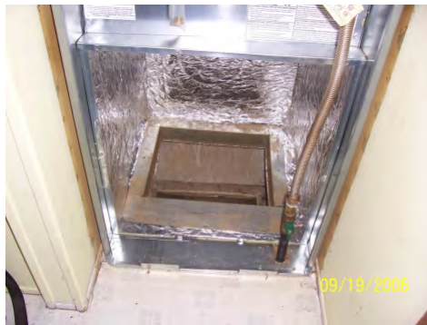
Remove the furnace panel. If the plenum to trunk connection is accessible here, complete sealing from this point
