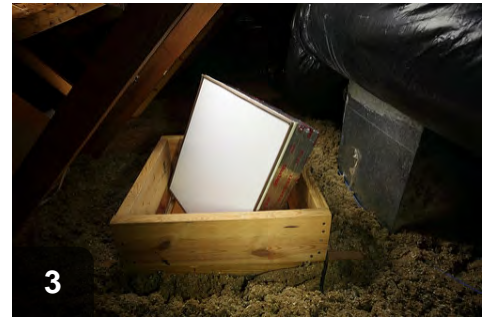
3 Weatherstrip around bottom edge of hatch cover to create air tight seal
