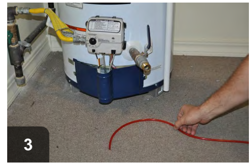
3 Place test hose by combustion appliance
