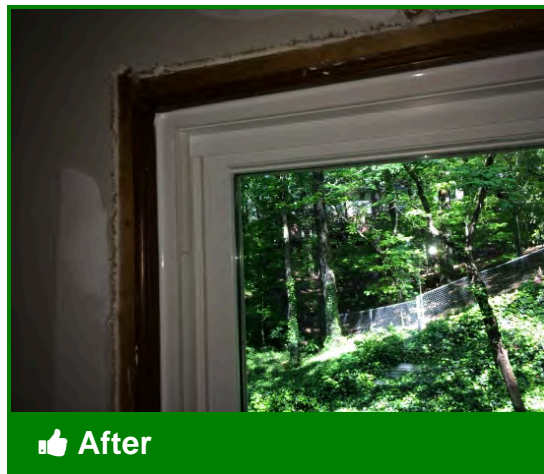
Replacement window installed, with stop molding replaced and caulked
