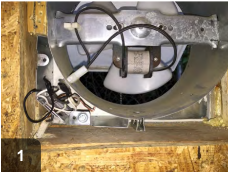
1 Inspect for: proper ground, wire nuts on splices, clamps on wiring where it enters junction box, cover installed on box
