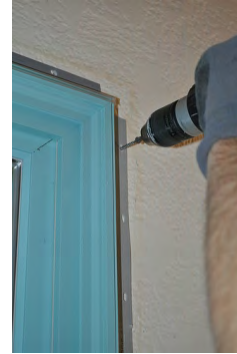
Fasten window flange securely around exterior of entire window
