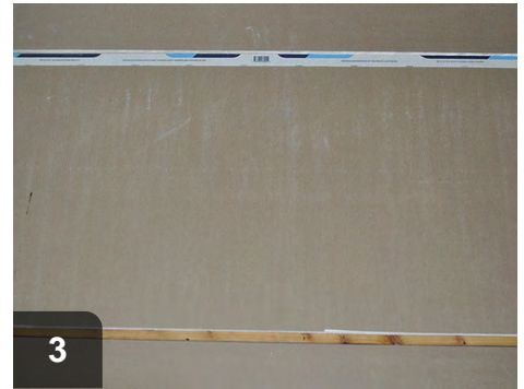
3 Cap soffit with rigid material, such as drywall, cut to size
