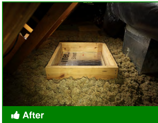
Hatch cover or panel access door should match r-value of attic insulation
