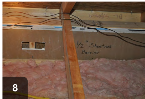
Drywall is also a good barrier for dense packing knee walls
