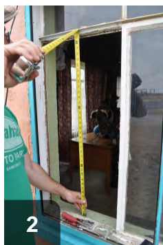
2 With broken glass removed, measure opening for replacement glass
