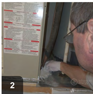
Seal penetrations around AC lineset and wiring
