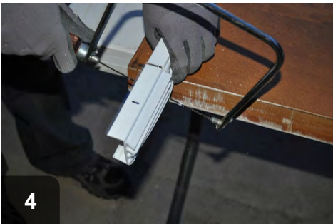
4 Cut door bottom to width of door
