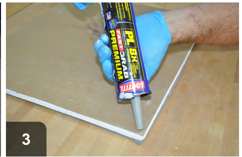
3 Apply strong adhesive to "cold-side" of hatch
