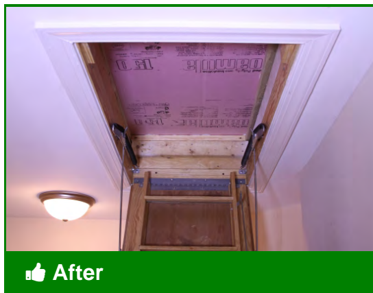
To preserve thermal envelope, an airtight seal needs to be created
