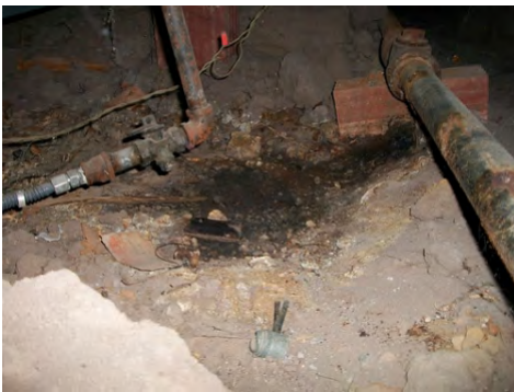
Any leaks found should be reported to occupant and work stopped
