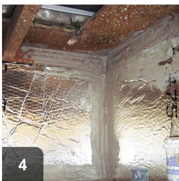
Seal all seams and joints with duct mastic
