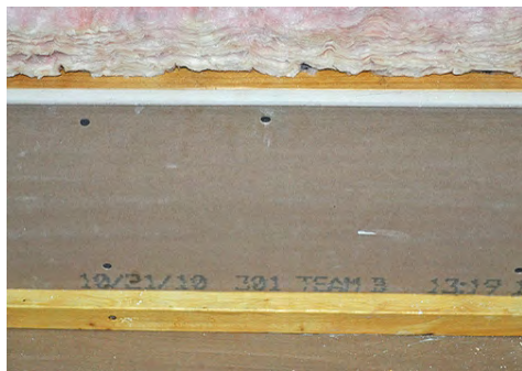
Option 3: Stud bay wall faced with rigid material, fastened and sealed
