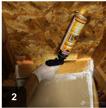
Carefully seal all seams and joints
