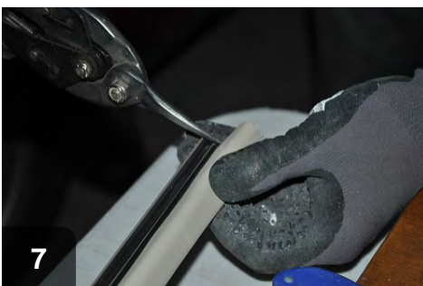
7 Notch upper ends of side weatherstripping to allow for top piece
