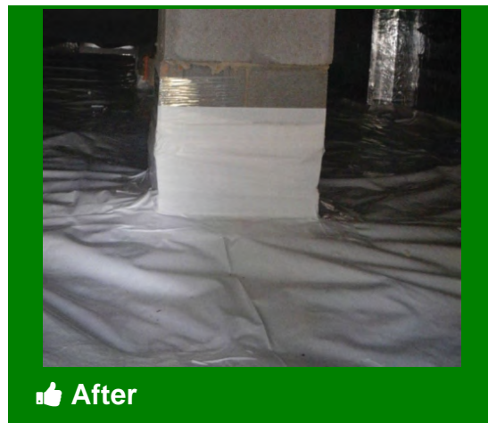
Ground moisture barrier should cover 100% of floor and at least 6" of walls
