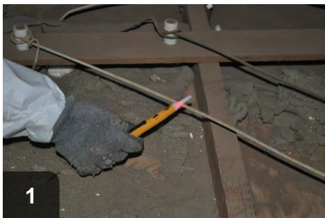
1 Have a certified electrician verify that wiring is safe to work around
