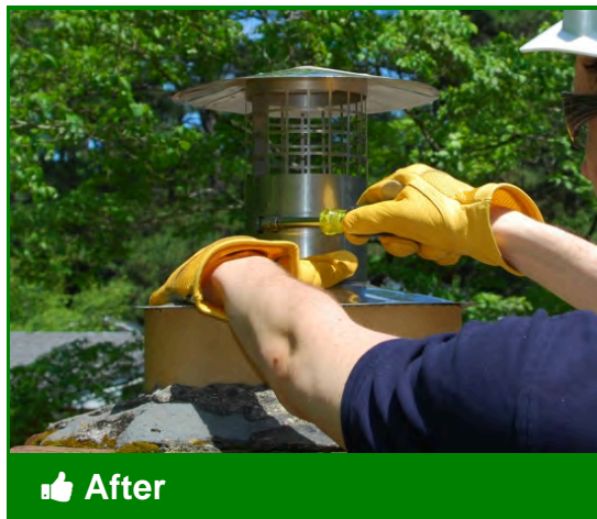
Flue liner with rain cap
