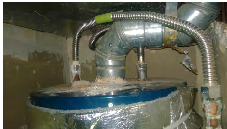
Inspect for missing draft diverter
