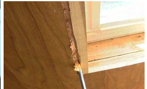
Fill interior gap with compressible foam or appropriate sealant
