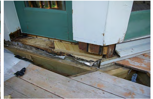
Cut new materials flush to surrounding surfaces and pitch toward exterior
