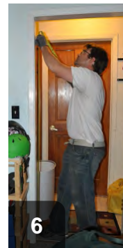
6 Measure doorway for weatherstripping
