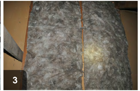
Batts should fill entire volume of knee wall stud bays
