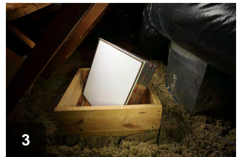
3 Weatherstrip underside of hatch cover to create tight seal
