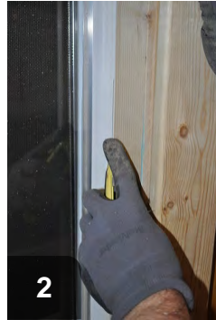
2 Cut through caulk at stops to break seal
