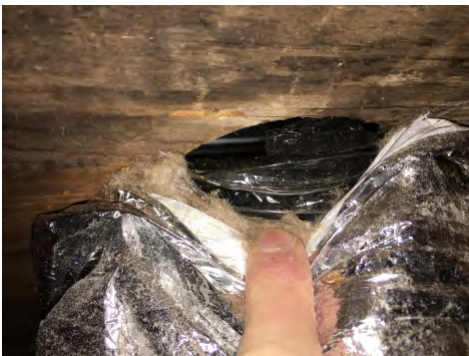
BAD/REWORK: Do not attach ducting to roof decking without a collar. A integrated collar must be used.
