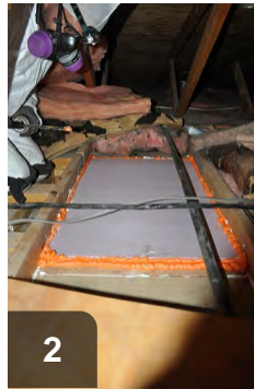
Use sealant to fill all remaining gaps
