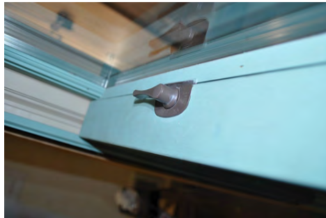
Check that sash locks align properly, indicating window is plumb
