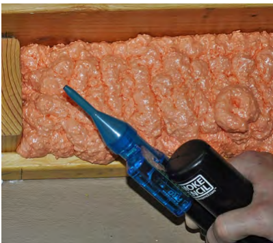
Whatever option chosen, test with chemical smoke to verify no leakage
