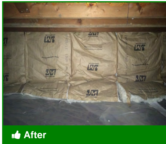
Batt insulation installed smooth, without gaps or voids, stapled in place
