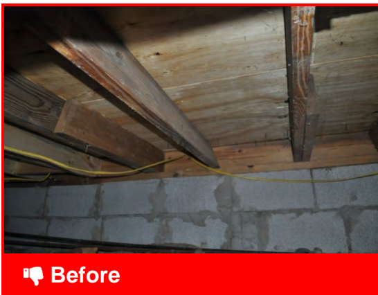
Uninsulated floors above unconditioned spaces are an energy drain
