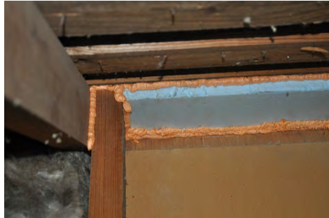
Top plate has been sealed to adjacent framing
