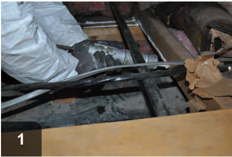
Apply sealant to surrounding surfaces before setting cap in place
