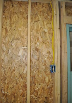
Open walls to be insulated and drywalled need air sealing
