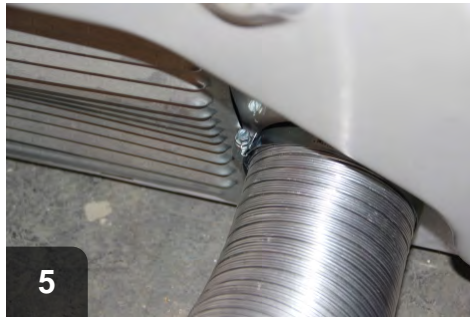
Connect vent pipe to dryer.
