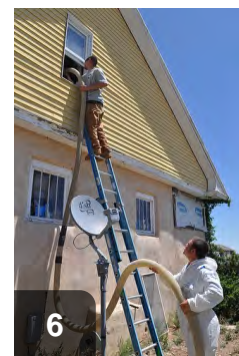
6 With dams in place, insulation can begin
