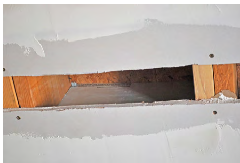
Rigid block will hold the insulation in place under the bonus room above
