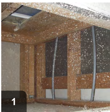
Identify building cavities used as ducts
