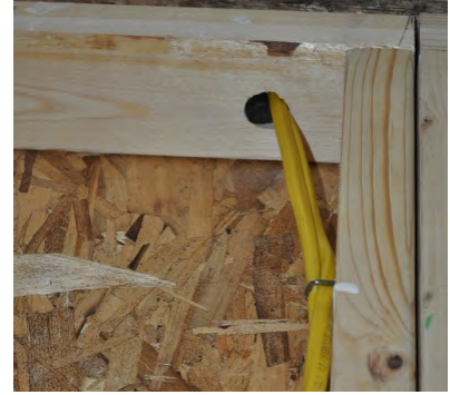
Use backer rod or other infill for larger penetrations
