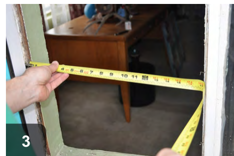
3 Cut replacement glass 1/8" smaller than measured opening
