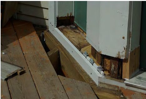
For exterior repairs, replace flashing
