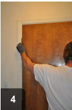
4 Rehang door to verify adjustments worked and door operates smoothly
