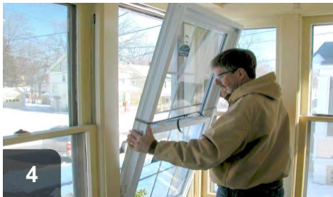
4 Apply caulk to stop molding and install the new window in accordance with manufacturer's instructions.
