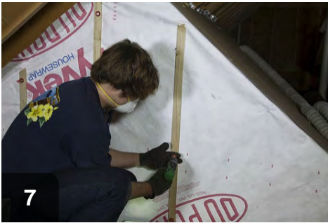
If using house-wrap or fabric, tack in place with furring strips or staples
