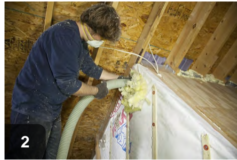
Insulation should meet manufacturer specifications for density.
