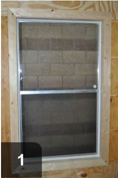
1 Single pane window needs to be replaced with double pane
