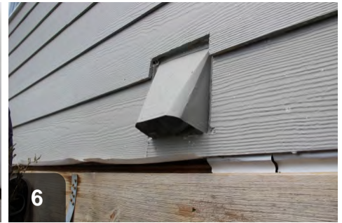
Dryer vents to outdoors, and exhaust damper is functional.
