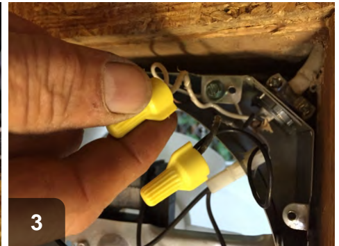
3 Install wire nuts on splices
