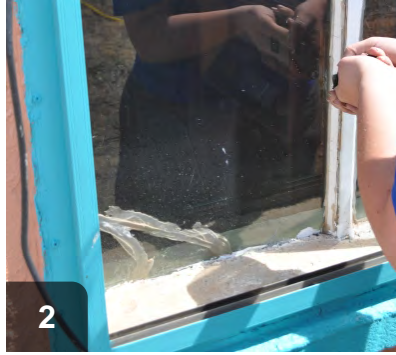
2 Cut through caulk bead and glazing to ease removal
