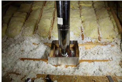
Dammed chimneys, flues and light fixtures prevent fires
