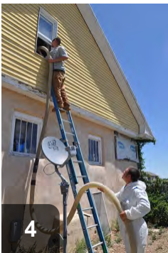
With modern wiring in place and old k&t disabled, insulation can begin
