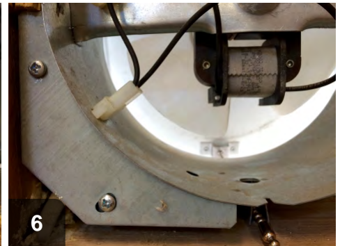
6 Reinstall cover on junction box
