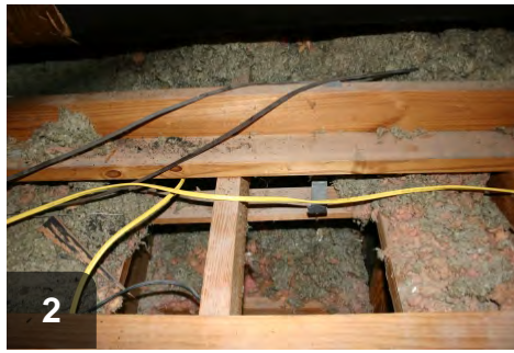
2 Clear away insulation and debris to allow inspection
