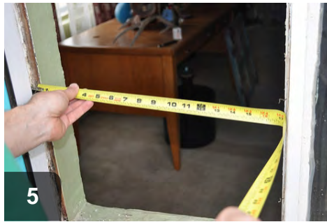
5 Cut replacement glass 1/8" smaller than measured opening
