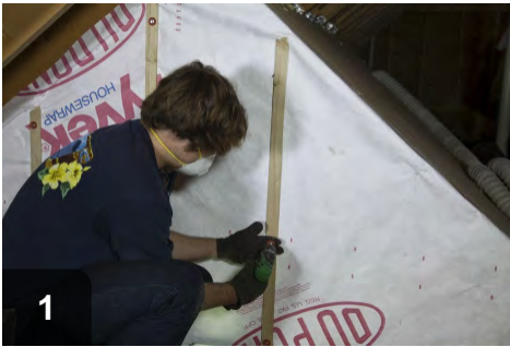
Attach furring strips to create pockets for dense-pack insulation
