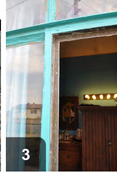
3 With sash cleaned, glass will fit properly and glazing will seal
