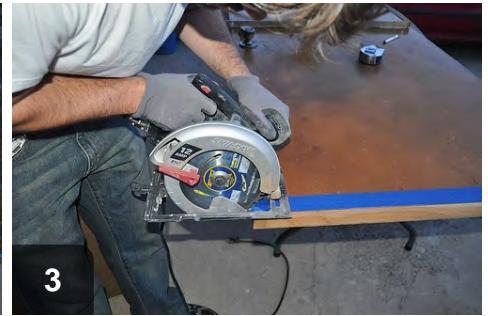
3 Trimming to allow for door bottom
