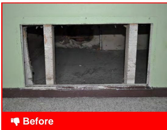
Leakage from air return into wall cavities should be eliminated
