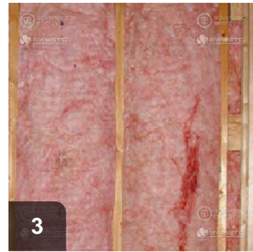
Install insulation in complete contact with all sides of the cavity.
