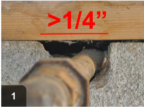
1 Measure holes to determine the best backing and fill strategy
