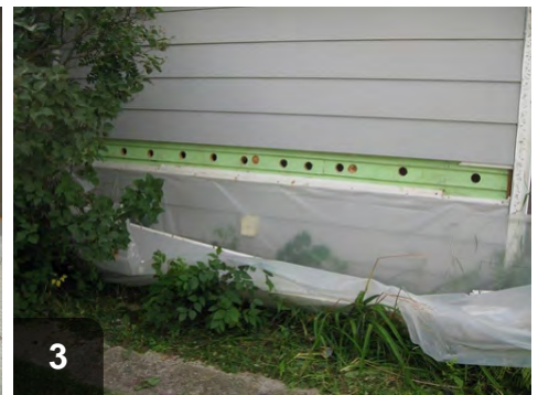
For exterior access, use a drop cloth or gutter to help with clean up
