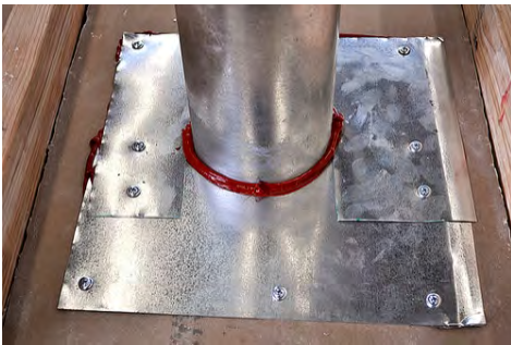
Only construct dam after sealing has been completed properly
