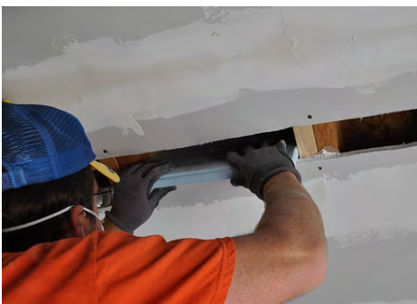
Rigid block should fit snugly into joist cavity to prevent insulation leaks
