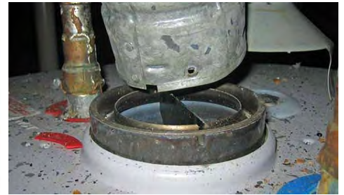
Inspect vent systems for disconnected pipes
