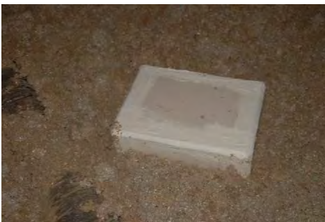
Non-IC can lights should be covered with a dam and have no insulation on top
