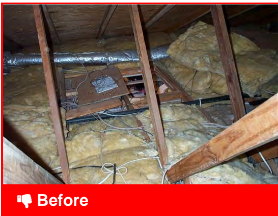
Uninsulated attic hatches and access panels weaken the thermal envelope
