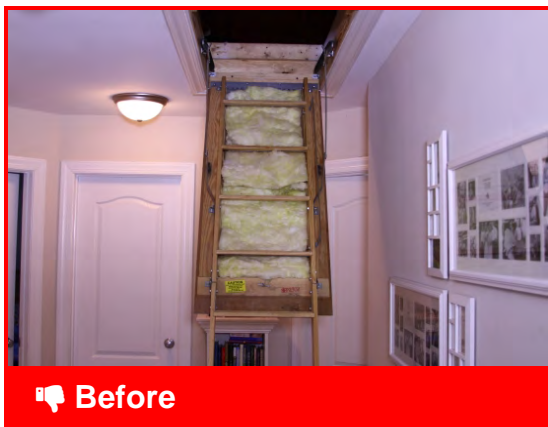
Unsealed pull-down stairs leads to air leakage to and from the attic
