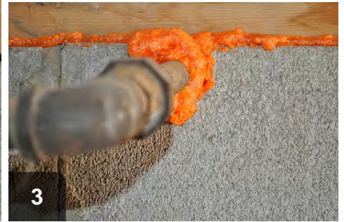
3 Sprayfoam or caulk seal the hole
