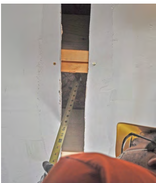
Measure joist cavity depth
