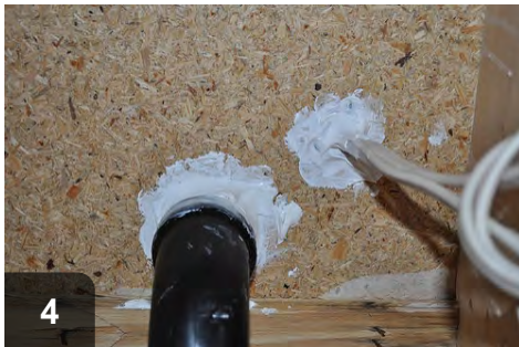
4 Visually inspect to verify no gaps remain
