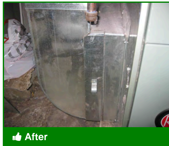
Filter slots should be covered
