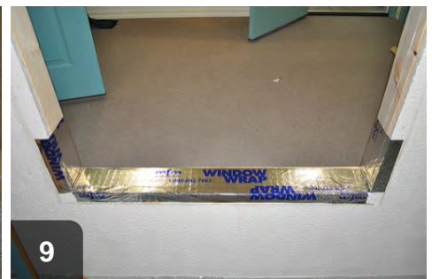
9 Install flashing along sides and bottom of rough opening
