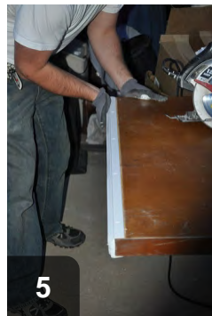
5 Ensure door bottom fits snugly around door and fasten into place
