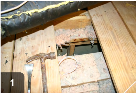
1 Locate and expose chases to prepare for inspection and capping/sealing
