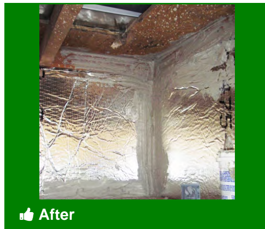
Return plenum lined with fiberglass duct board and sealed with mastic
