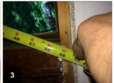
3 Measure diagonally both ways across opening. If measurements are equal, the opening is square
