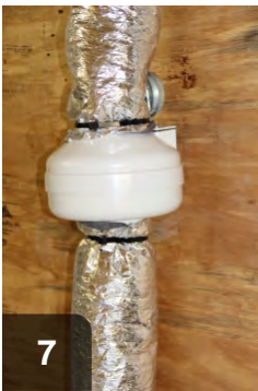
For vent runs >35 feet, a booster fan is required.
