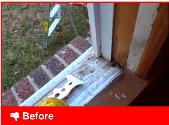
Window opening ready to receive replacement window
