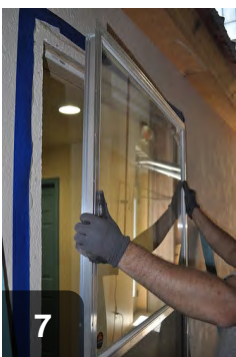
7 Remove window from rough opening
