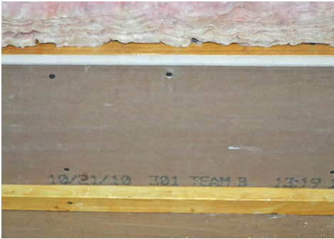
Sealing with drywall reduces overall combustibility of paneled chases
