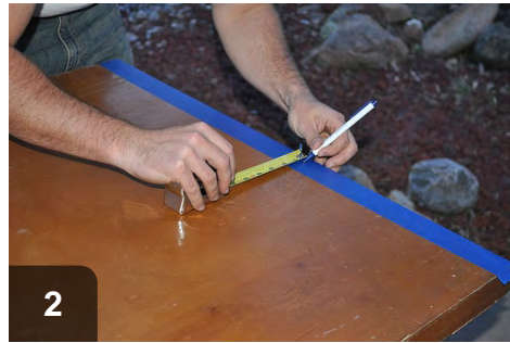
2 Measure and trim door, if necessary, to allow for door bottom
