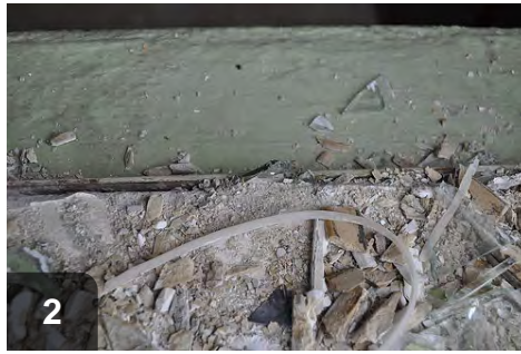
2 Check closely to remove all pieces of broken glass and debris
