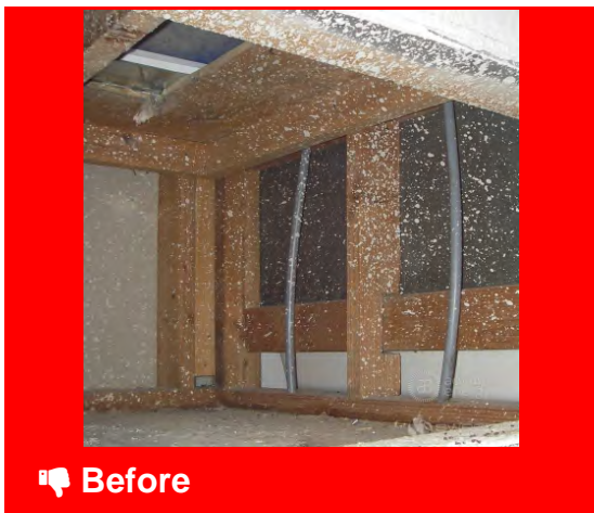
Locate unsealed ducts constructed from building cavities
