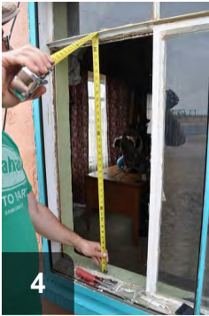
4 With points and glass removed, measure opening for replacement pane
