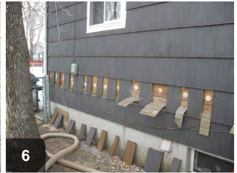
6 If possible, maintain house wrap, or replace it after holes are plugged
