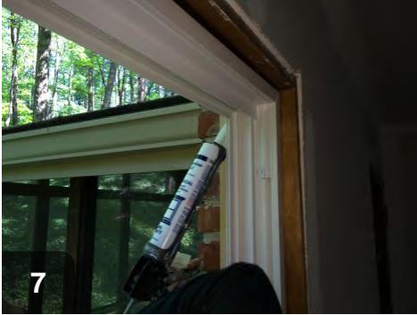
Caulk new window to existing stop molding
