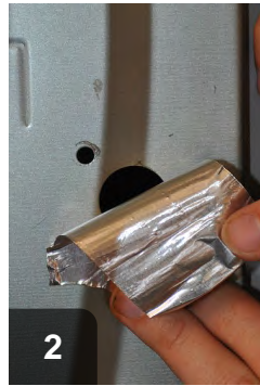
Removable foil tape should be used to seal
