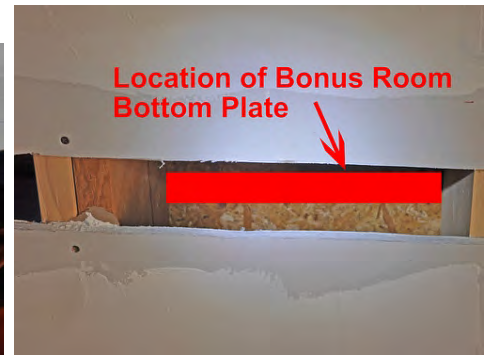
The rigid block should be placed in line with the stem wall above
