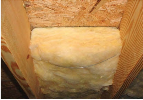
Batt should be in contact with subfloor without being compressed
