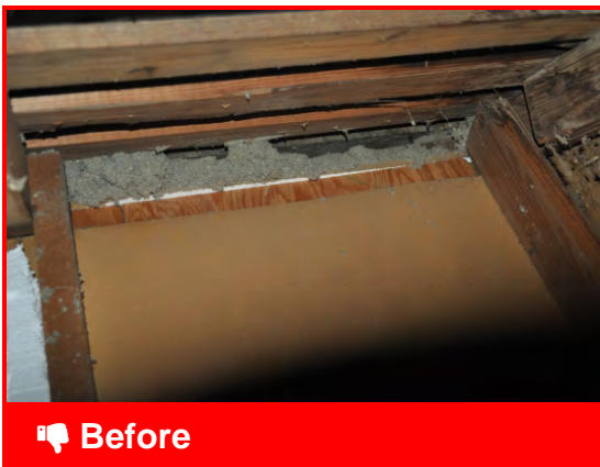
Top plate is missing from knee wall
