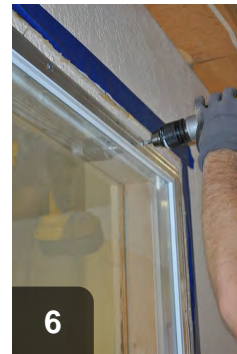
6 Remove exterior fasteners to free window
