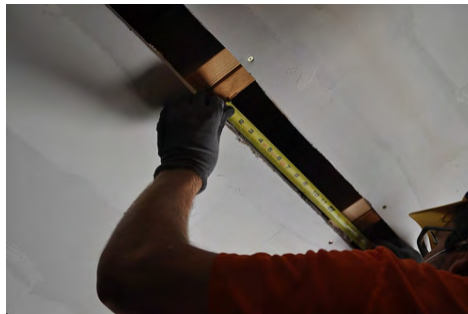
Measure joist cavity width
