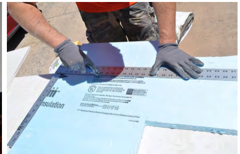
Cut XPS, or other rigid material, to measured size of joist cavity
