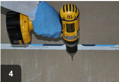
4 Fasten cap with screws to set sealant and create air barrier
