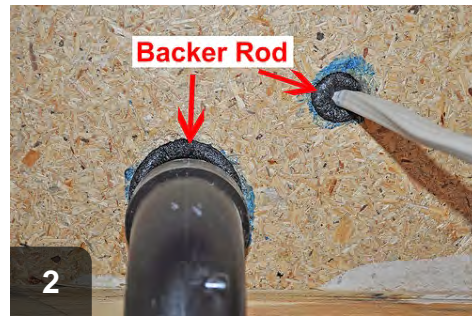
2 Infill with backer rod
