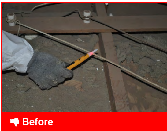
Knob & tube wiring needs to be tested to determine if still live. Red=live
