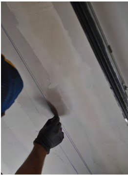
Snap chalk lines to keep access cuts clean and easy to repair
