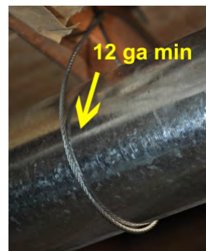
Metal wire should be at least 12 gauge and galvanized
