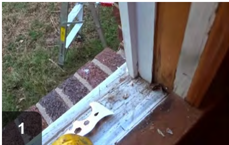
1 Prepare and clean opening before installing new window
