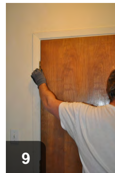
9 Rehang door and verify fit, operation, and lack of air infiltration
