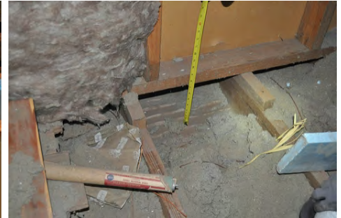
Bottom plate is also missing. Space is measured so XPS can be cut
