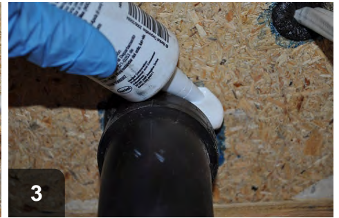
3 Apply appropriate caulking to ensure backing/infill does not move
