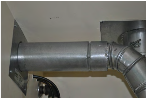
Inspect vent systems for inadequate slope
