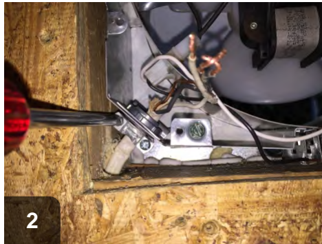
2 Install clamp on wiring into junction box
