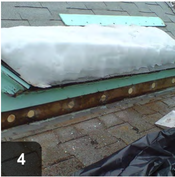
4 Plug holes with rigid material that will not move or sag over time
