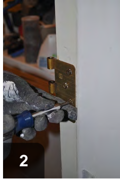
2 Adjust hinge plates to bring door back into true
