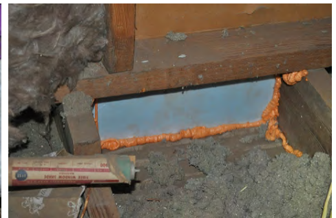
Bottom plate is also sealed to surrounding joist and framing
