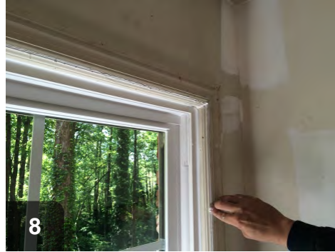
Reinstall and caulk interior stop molding
