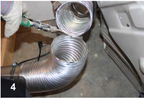
Trim metal vent to ensure the run is as short and straight as possible.
