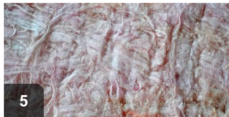
5 Insulate over now-capped soffit
