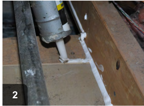
Sealant should extend along joists and into seams at top plates
