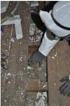
Check cavity for electrical junction and penetrations
