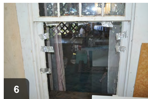
6 Secure pane in place with tape to hold until glazing sets
