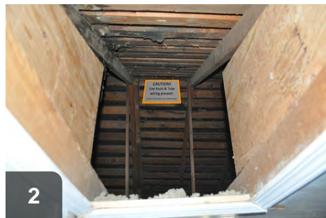
2 A sign should be posted at all entrances to warn of knob & tube wiring
