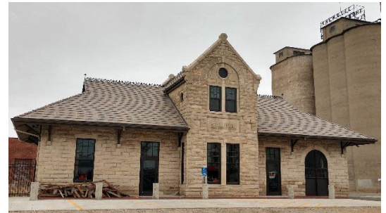
NCRPC administered a CDBG Commercial Rehabilitation project that helped restore a former depot on North Santa Fe Avenue in Salina.
