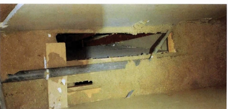
TWIN VALLEY APARTMENTS ATTIC PICTURES (14)
