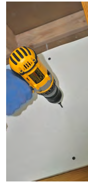
Bracing can be screwed to drywall before capping chase
