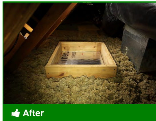
Once sealed, air leakage at attic hatch or door should be minimized
