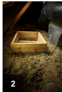
2 Build dam to hold back attic insulation and hold cover in place tightly
