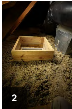
2 Build insulation dam from 3/4 inch lumber and seal around base
