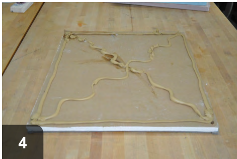
4 Adhesive should ring perimeter as well as criss-crossing hatch to ensure complete attachment of insulation
