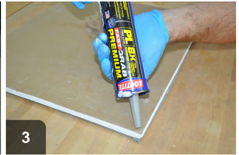
3 Apply strong adhesive to "cold-side" of hatch
