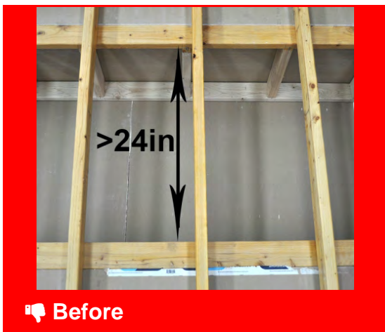
Spans greater than 24 inches require additional bracing before capping
