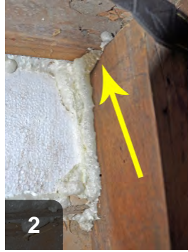
Extend seal along adjacent framing
