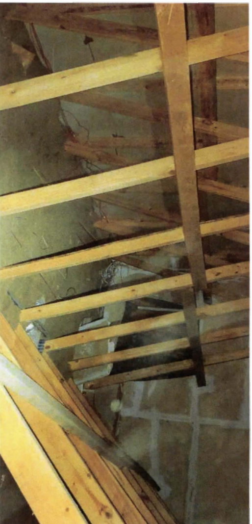
TWIN VALLEY APARTMENTS ATTIC PICTURES (INSULATION) (1)
