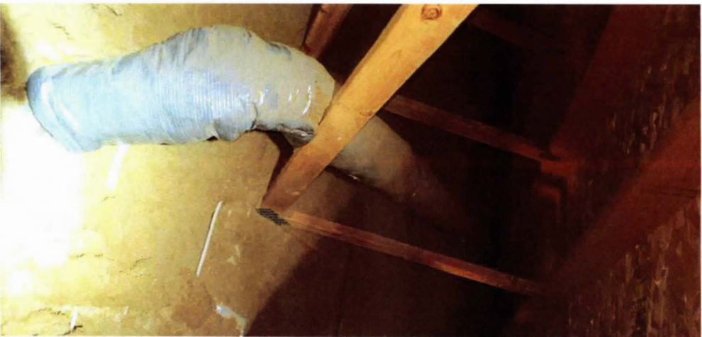
TWIN VALLEY APARTMENTS (RANGE HOOD DUCT RAN TO SOFFIT) (1)
