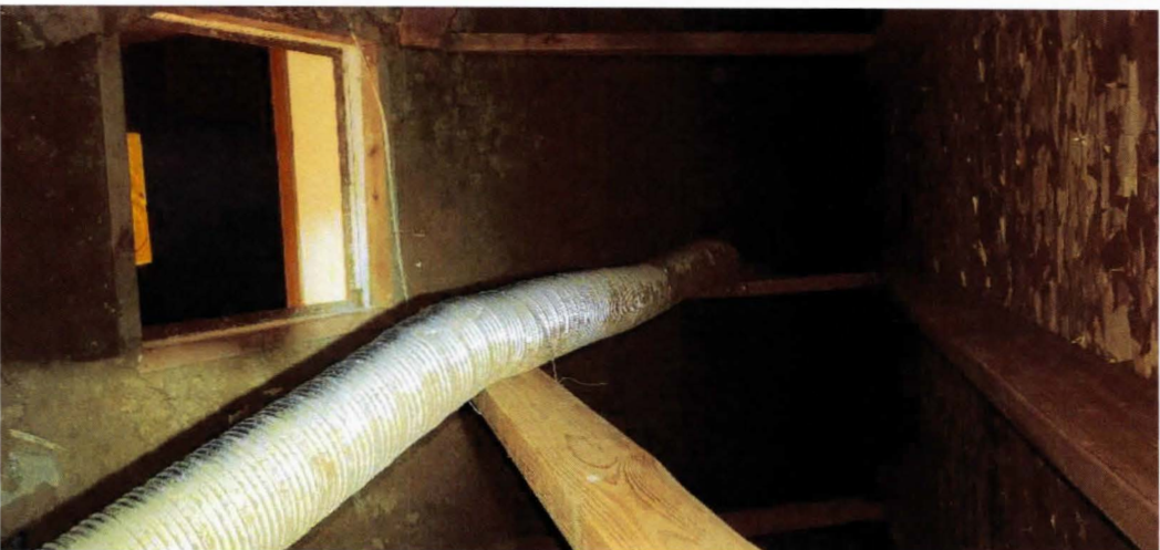
TWIN VALLEY APARTMENTS (EXISTING BATH FAN DUCT - RAN TO SOFFIT)
