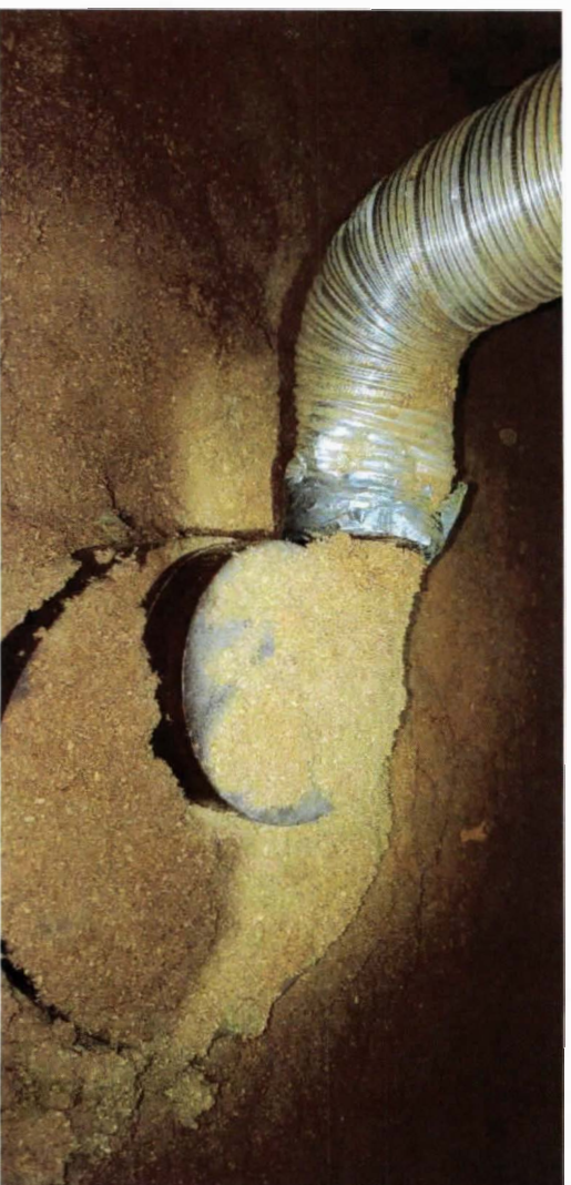
TWIN VALLEY APARTMENTS ATTIC PICTURES (BATH FAN) (1)
