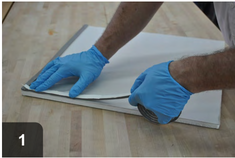
1 Apply foam tape to "warm side" face of attic hatch
