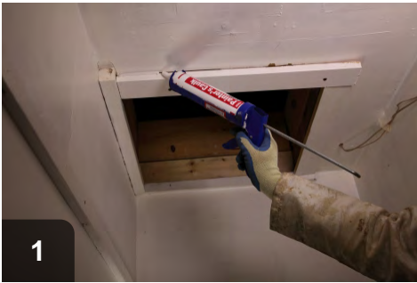
1 Remember to seal around finish details and framing on interior
