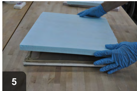
5 Affix XPS insulation to "cold-side" of hatch with adhesive, ensuring XPS is tight and square to hatch
