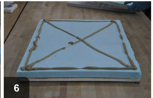
6 Repeat adhesive and XPS layers to reach maximum R-value without making hatch excessively heavy or awkward
