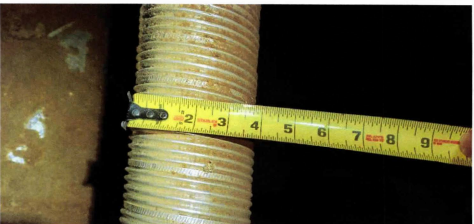
TWIN VALLEY APARTMENTS ATTIC PICTURES (BATH FAN DUCT) (2)
