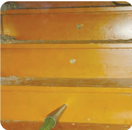
10. If backside of stairs is sealed, blow insulation into cavity behind stairs
