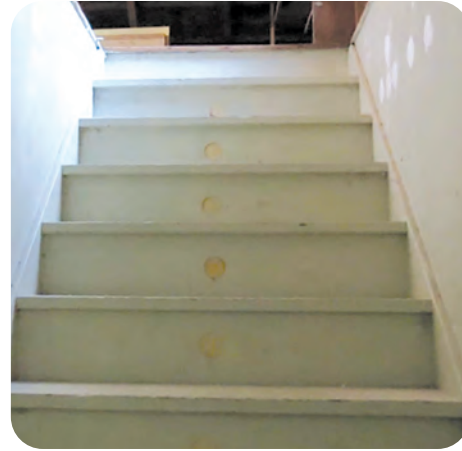
11. Plug access holes from blown insulation
