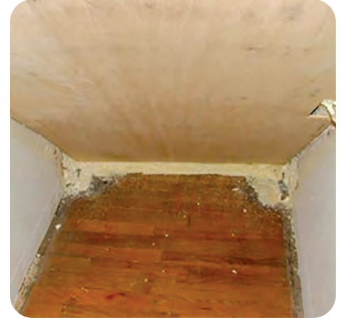
9. Insulate under stairway and seal off insulation from conditioned space in home
