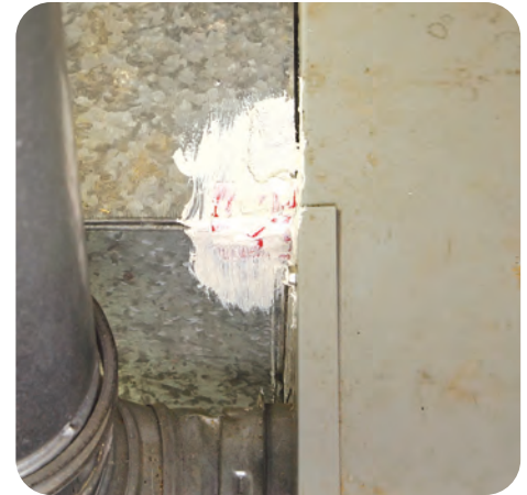
B-3. Apply mastic over the tape
