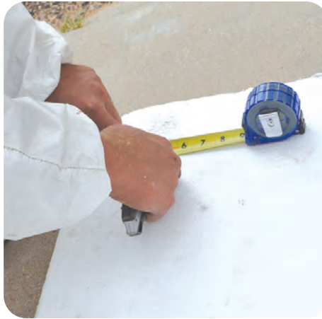
2. Cut blocking material to fit
