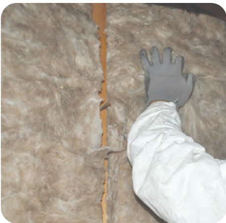
3. Install batts with minimal compression
