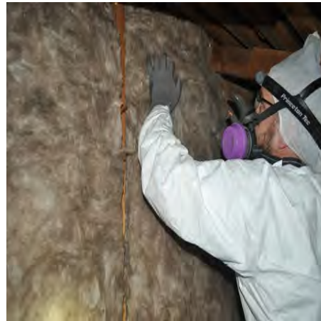
4. Kraft-face should go to "warm in winter" side and batt should fill the entire bay for a grade 1 installation.
