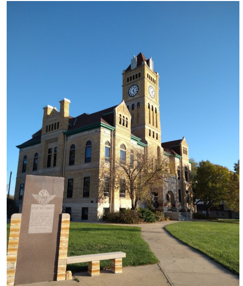
Mitchell County utilized the State Historic Rehabilitation Tax Credit Program for an exterior restoration project on its courthouse this year. (Photo courtesy of Doug McKinney)
