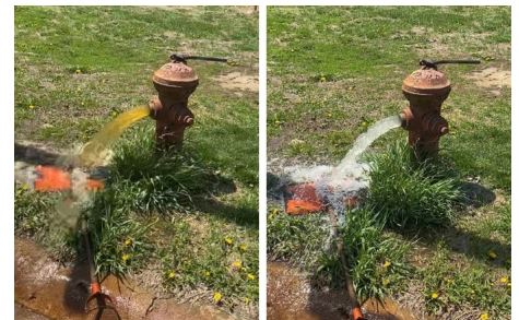
Top Photo: A two-phase project in the City of Vermillion is working to resolve many water issues, including the presence of sludge filled/corroded pipes. (Courtesy Photo)
