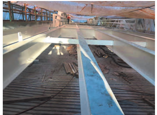
4. Green Bridge – Historic Pony Truss Rehabilitation
