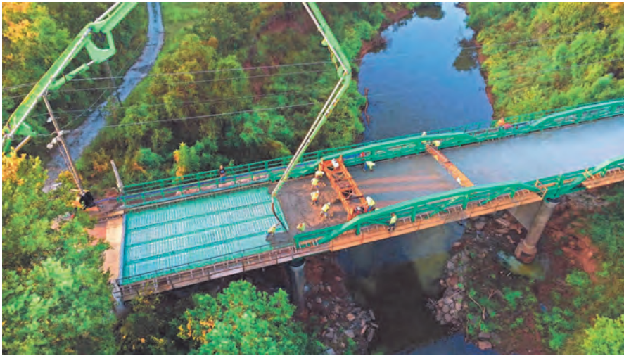
Green Bridge – Historic Pony Truss Rehabilitation
