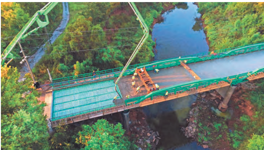
4. Green Bridge – Historic Pony Truss Rehabilitation
